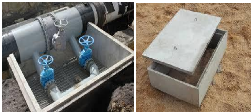
Plate 2.3 Typical Valve Pit
