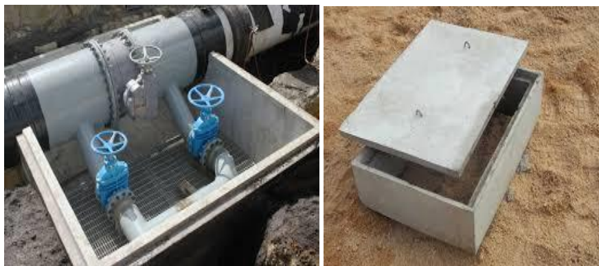
Plate 2.3 Typical Valve Pit
