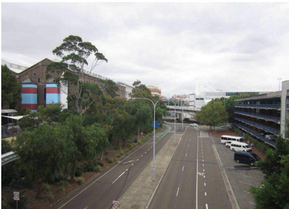
Figure 48 Looking north along Darling Drive and the Rail Corridor – Powerhouse museum to left, Entertainment Centre carpark to right.
