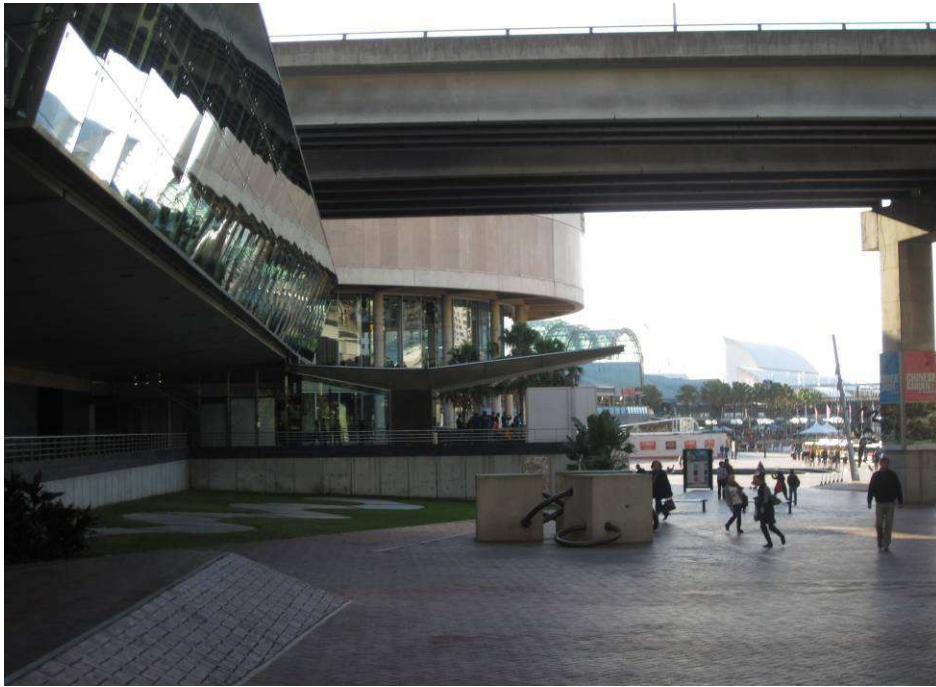
Figure 27 Looking north from the 1999 link building.
