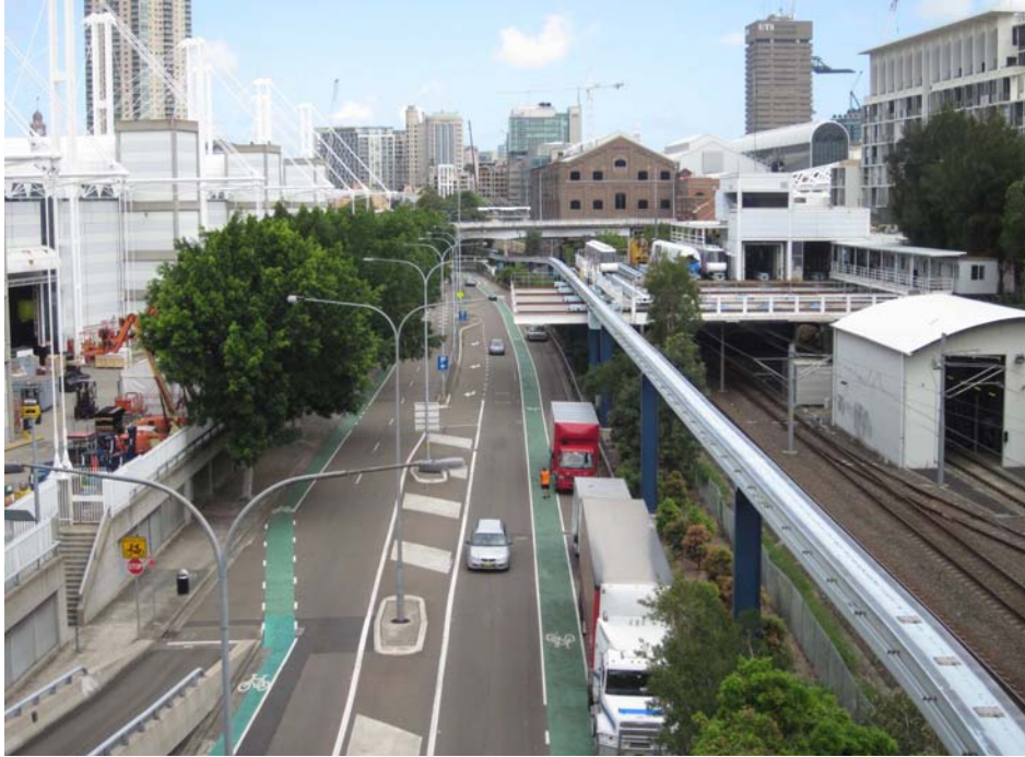
Figure 43 Darling Harbour Rail Corridor looking south from the M4 overpass. Monorail infrastructure spans the Darling Harbour Rail Corridor.
