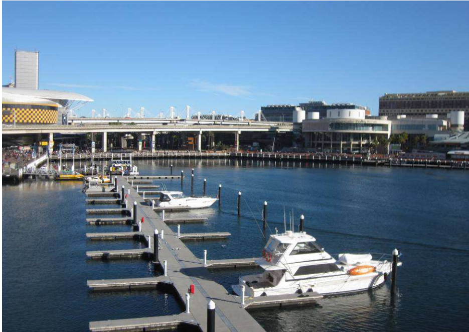
Figure 23 Convention Centre viewed from Pyrmont Bridge. The structure of the Exhibition Centre can be seen beyond the M4 overpass.
