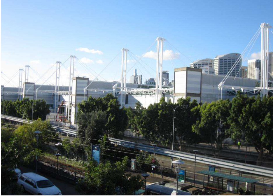
Figure 41 Exhibition Centre viewed from the southwest.
