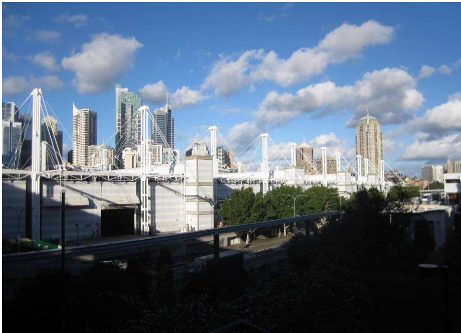
Figure 42 Exhibition Centre viewed from the northwest.
