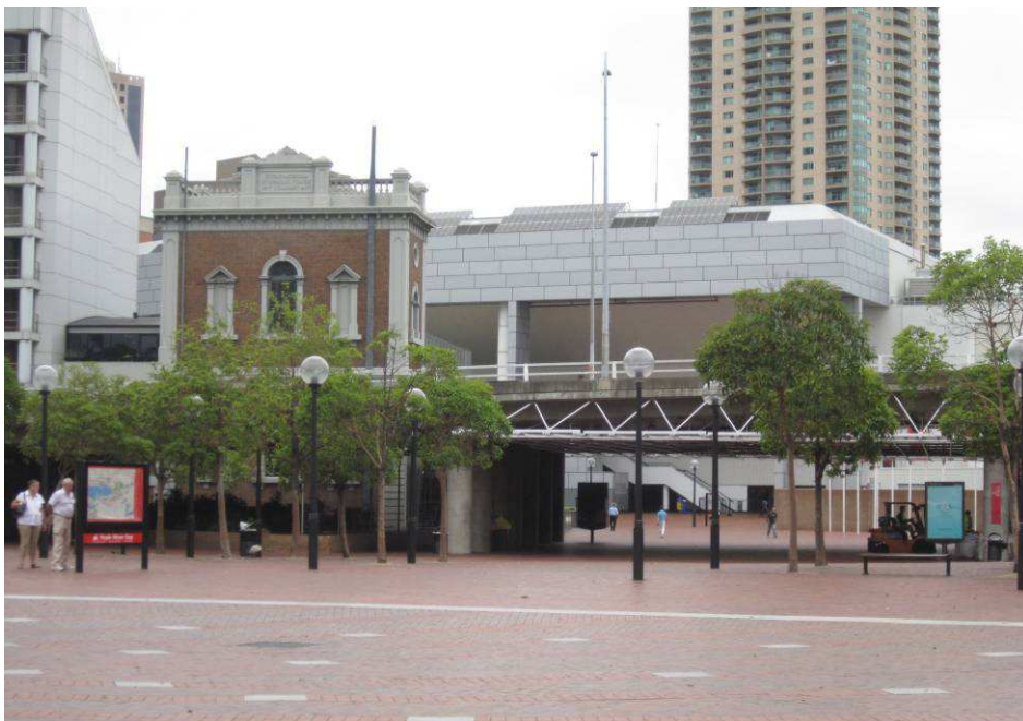
Figure 52 Hydraulic Pumphouse and Entertainment Centre viewed from the north.
