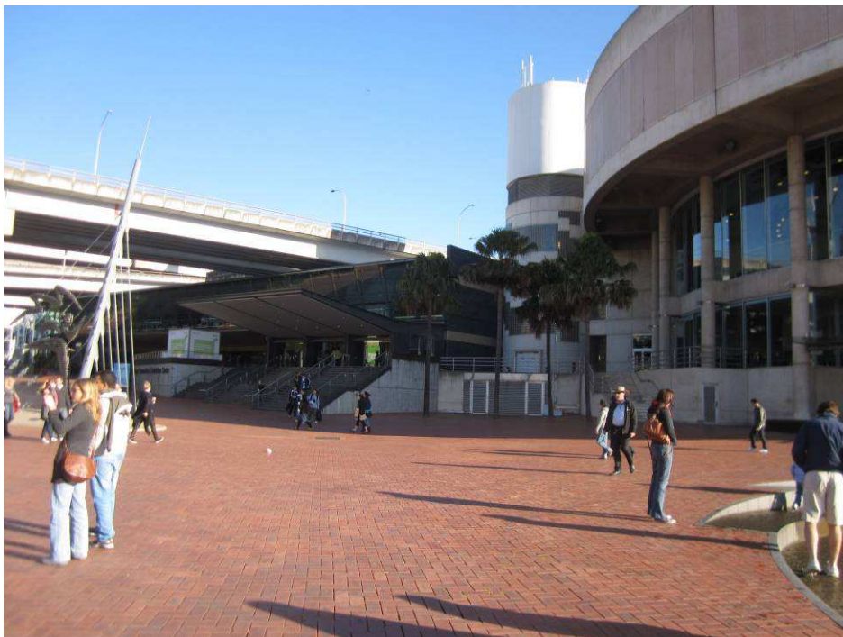
Figure 26 Looking south from the Convention Centre towards the 1999 link building and the M4 overpass.
