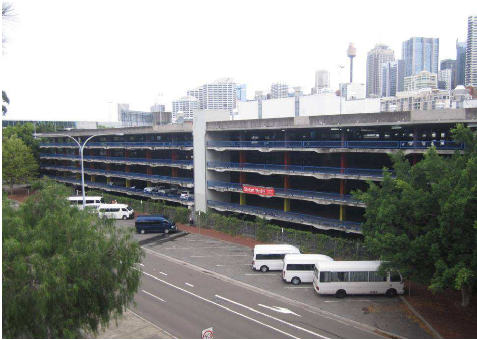
Figure 49 Entertainment Centre carpark.
