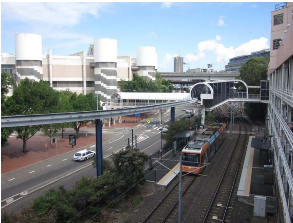
Figure 28 Western side of the Convention Centre, monorail infrastructure and pedestrian links to the Novotel.
