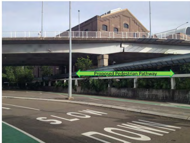
Pedestrian path to west of Darling Drive
