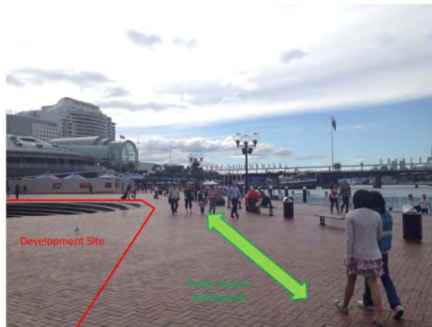
Concourse access around hoarding line
