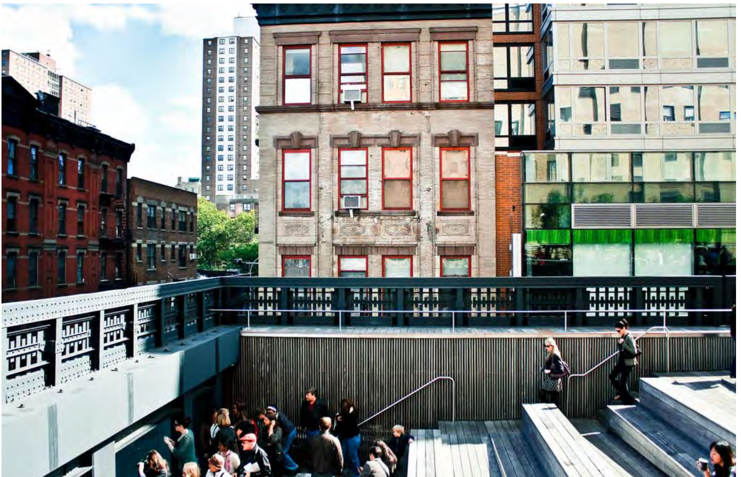
THE HIGH LINE, NEW YORK CITY: CREATIVE SEATING SPACE WITH DDA COMPLIANT ACCESSIBLE ACCESS TO THE VIEWING WINDOW
