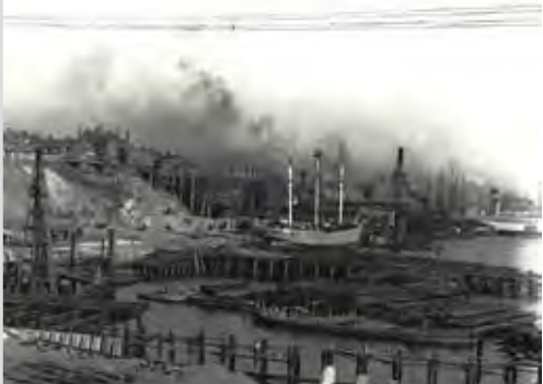
VIEW OF THE RECONSTRUCTION OF DARLING HARBOUR FROM MILLERS POINT SHOWING DALGETYS WHARF NO.1 PARTLY COMPLETED. DATED: 1909 DIGITAL ID: 9856_A017_A01700007
