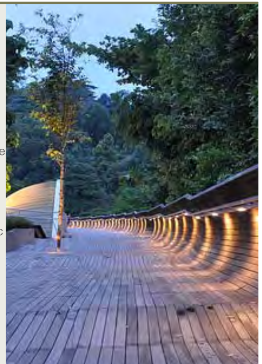
GARDEN CITY PEDESTRIAN BRIDGE, SINGAPORE
