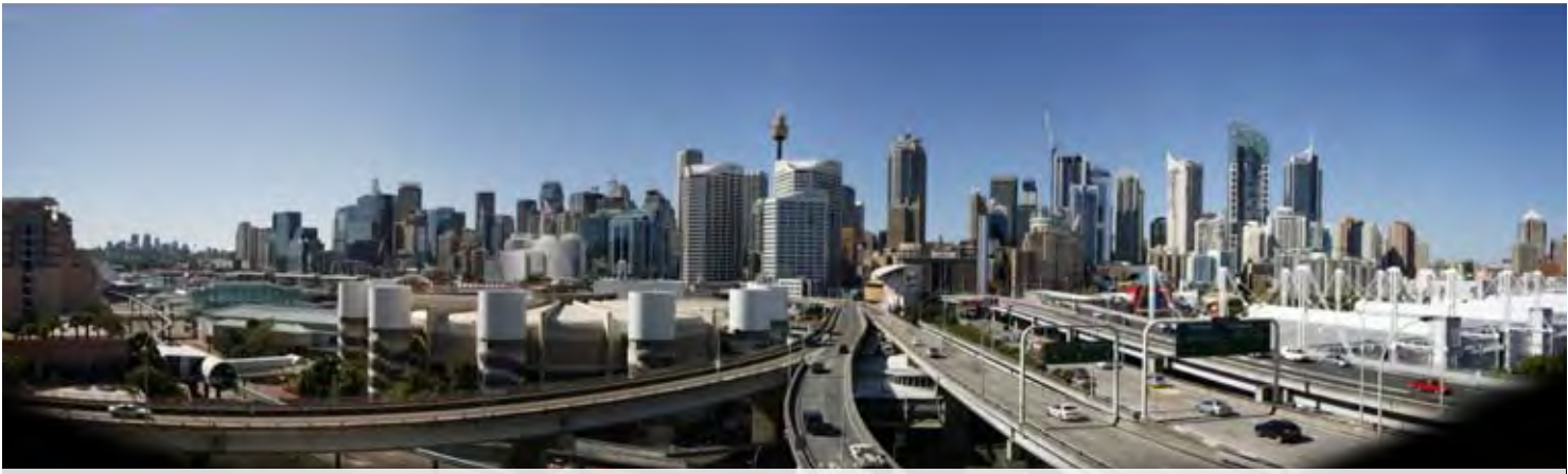
EXISTING CONVENTION CENTRE, WESTERN DISTRIBUTOR AND EXHIBITION CENTRE, DARLING HARBOUR, VIEW TO EAST
