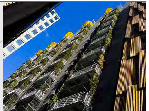
CH2 BUILDING MELBOURNE; EXPRESSES ITS ENERGY AND RESOURCE CONSUMPTION
