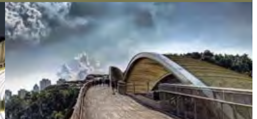
ELEVATED TIMBER DECK THROUGH THE CANOPY
