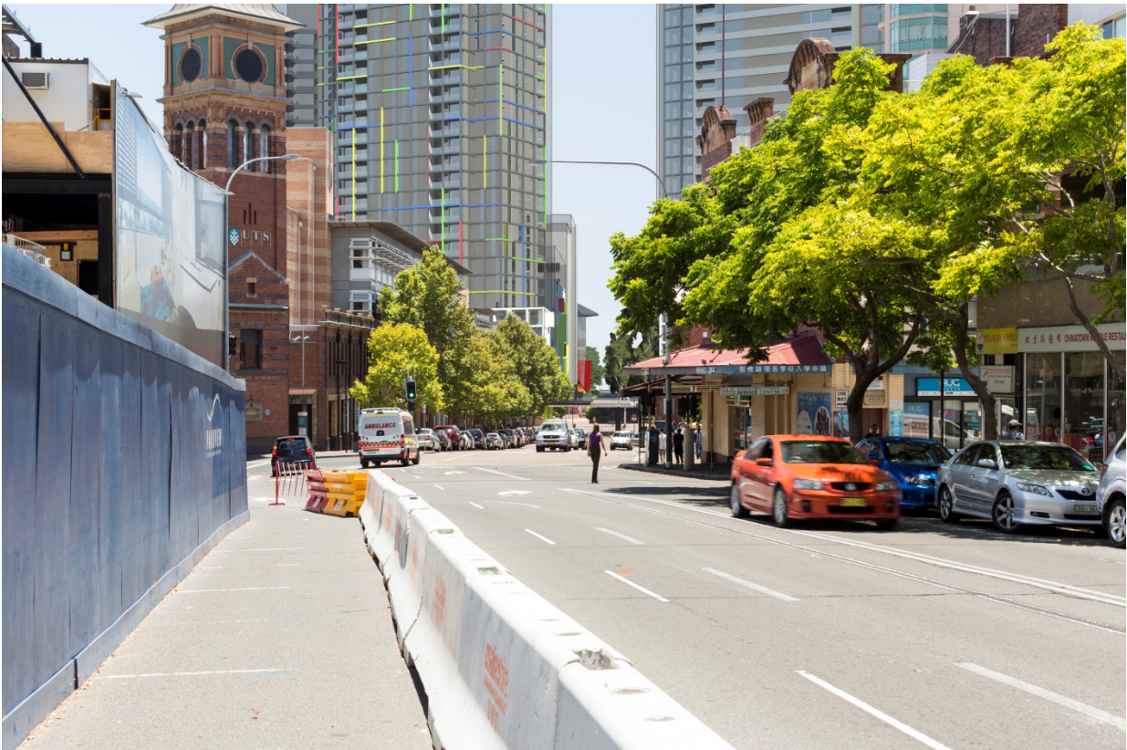
SICEEP Ground View Corridor 24
