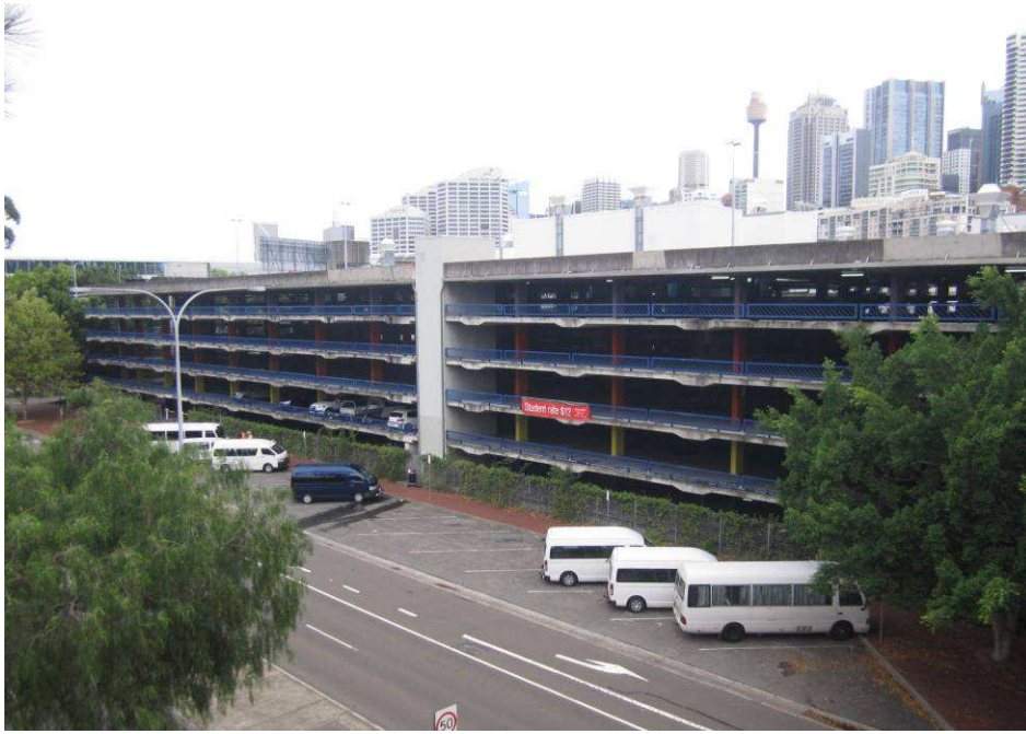
Figure 50 Entertainment Centre carpark.
