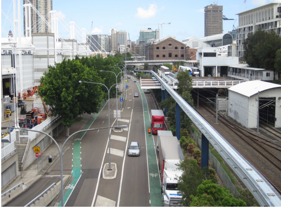
Figure 44 Darling Harbour Rail Corridor looking south from the M4 overpass. Monorail infrastructure spans the Darling Harbour Rail Corridor.
