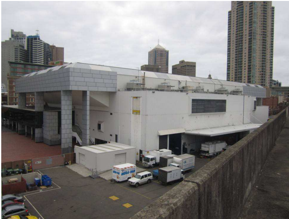
Figure 54 Entertainment Centre viewed from the northwest.
