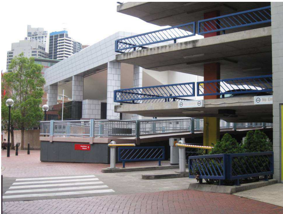
Figure 51 Looking east from the Entertainment Centre carpark towards the Entertainment Centre.
