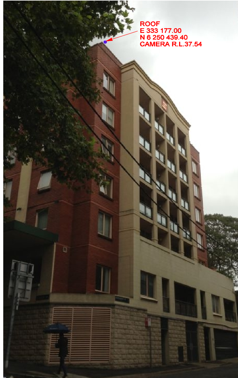
No.318 HARRIS STREET PYRMONT
