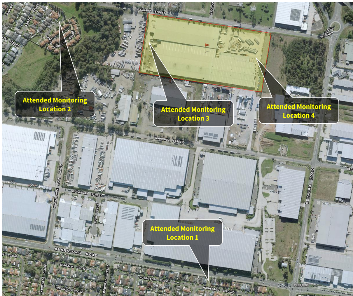
Figure 1. Subject site and monitoring locations – Image sourced from Six Maps
