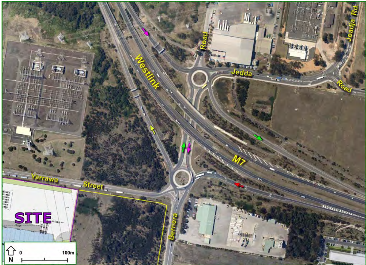
Figure 6: Westlink M7 / Bernera Road Interchange
