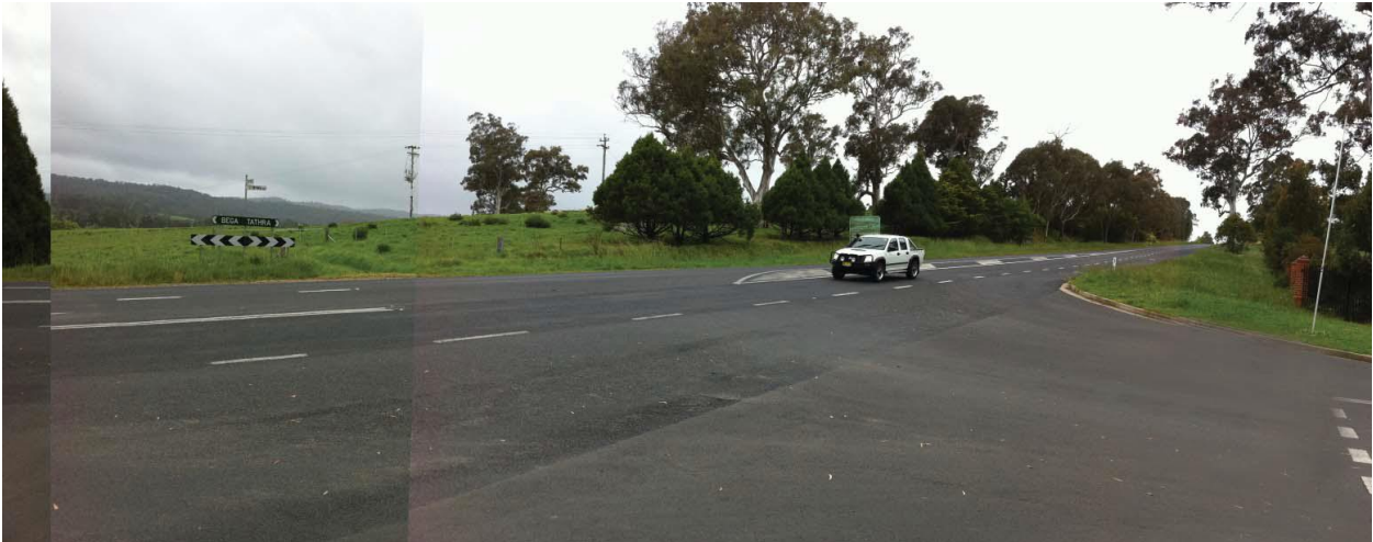
FIGURE 1 – LOOKING EAST/SOUTH FROM INTERSECTION OF TATHRA ROAD AND HARRY SCANES AVE
