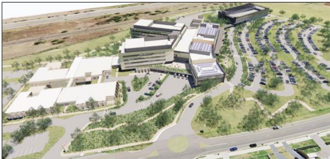
Figure 1: Aerial Perspective of NSH from Entry on Dunmore Road (COX+STH 2023)
