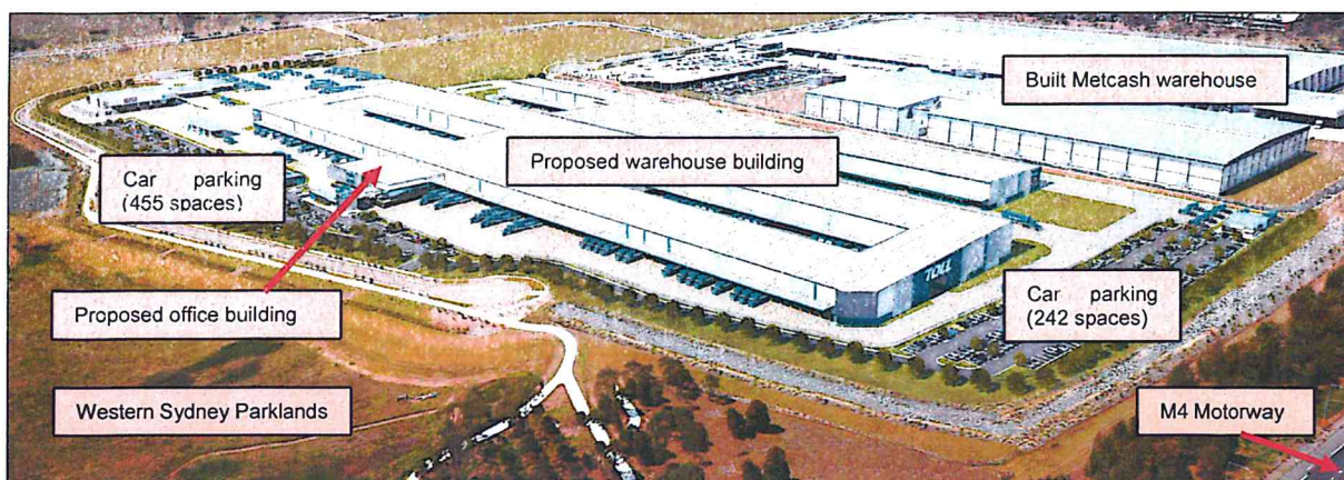
Figure 3 – Site layout, view north east
