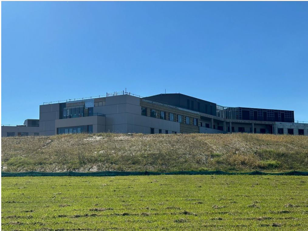
Photo 1: Main Building Construction
