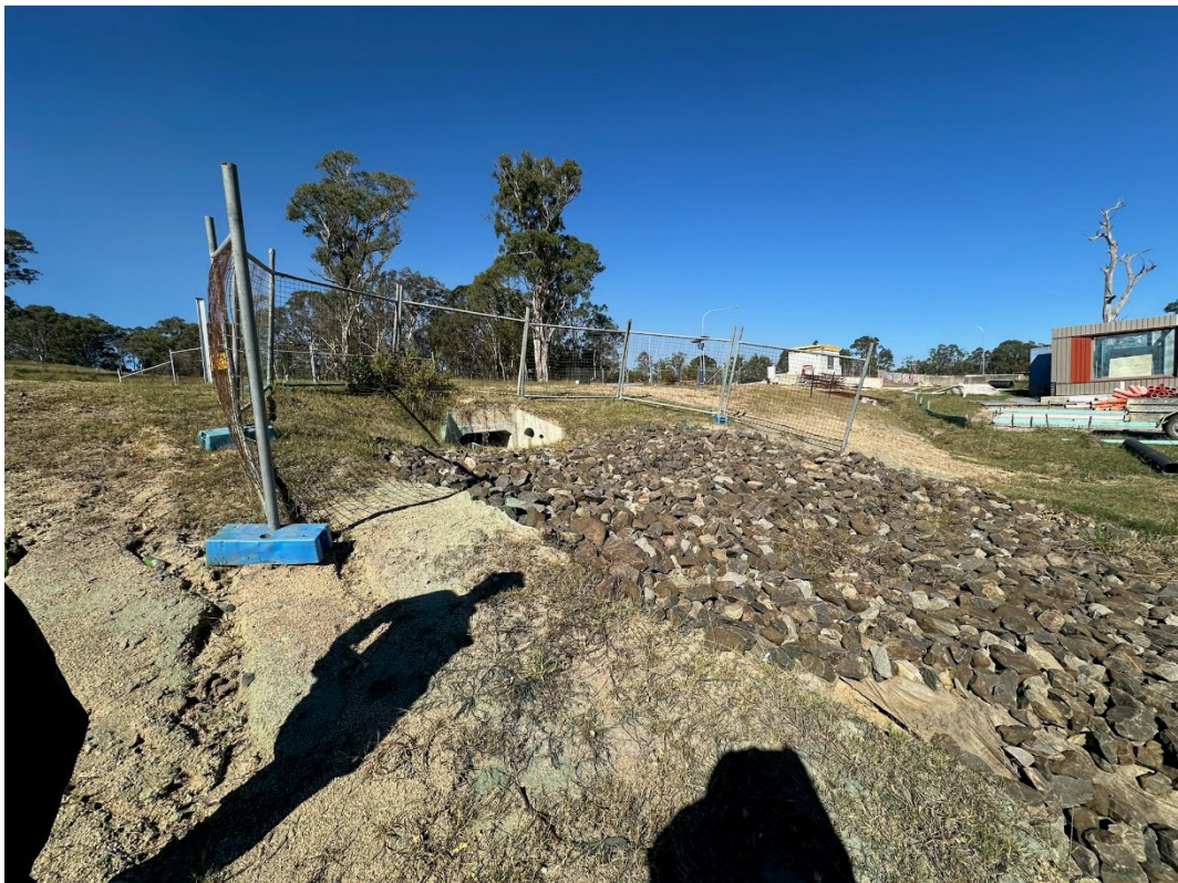
Photo 4: Final drainage works
