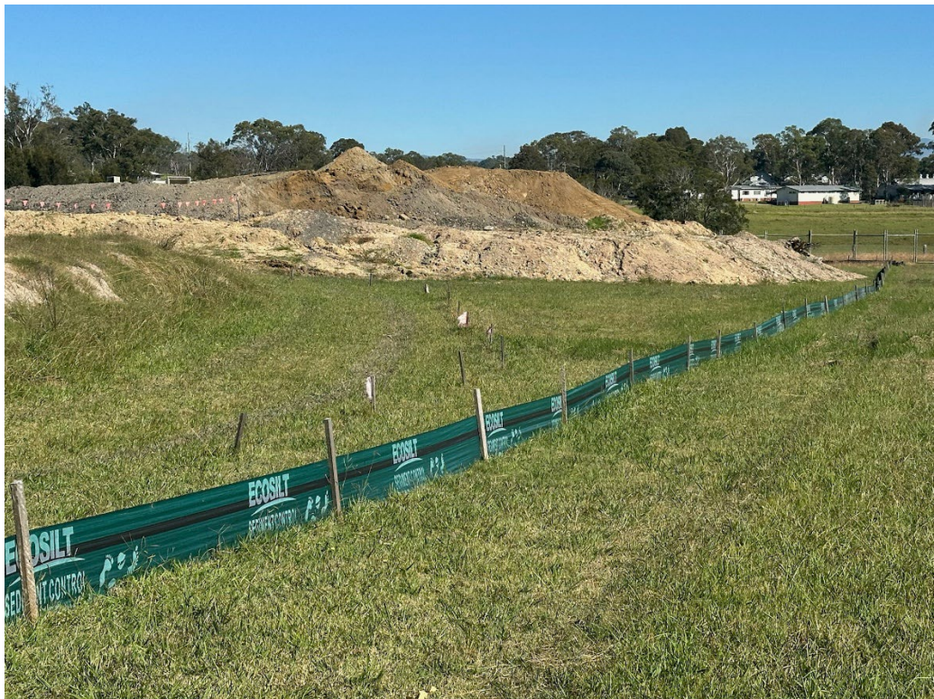
Photo 6: Silt fence surrounding spoil stockpile
