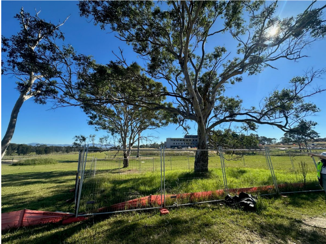
Photo 9: Tree protection fencing
