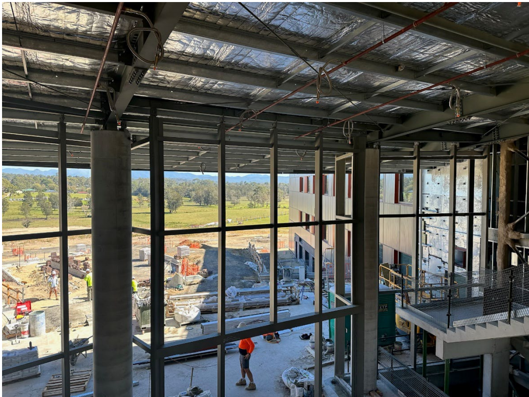
Photo 3: Internal fitout and glass facade
