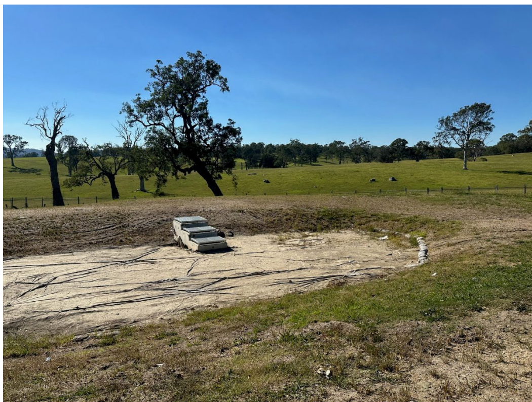
Photo 8: Operational sediment basin
