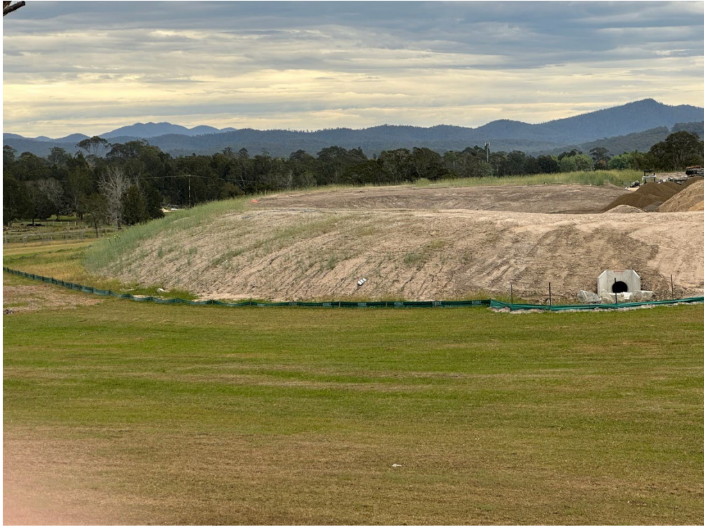
Photo 7: Earthworks batter shaped and formed
