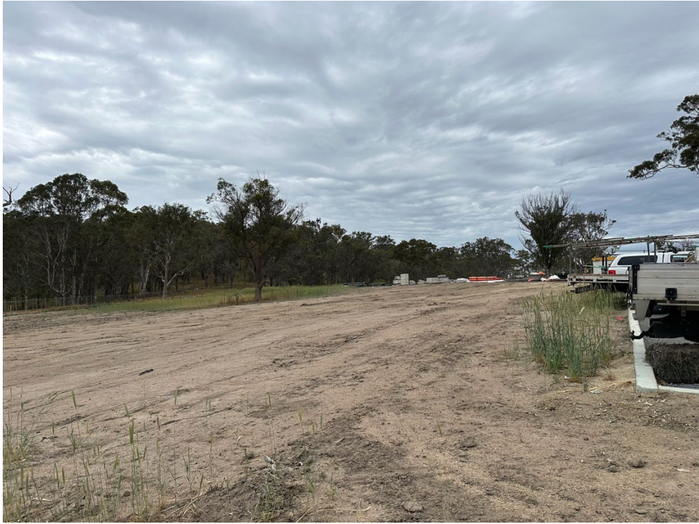
Photo 13: Exposed area subject to stabilisation
