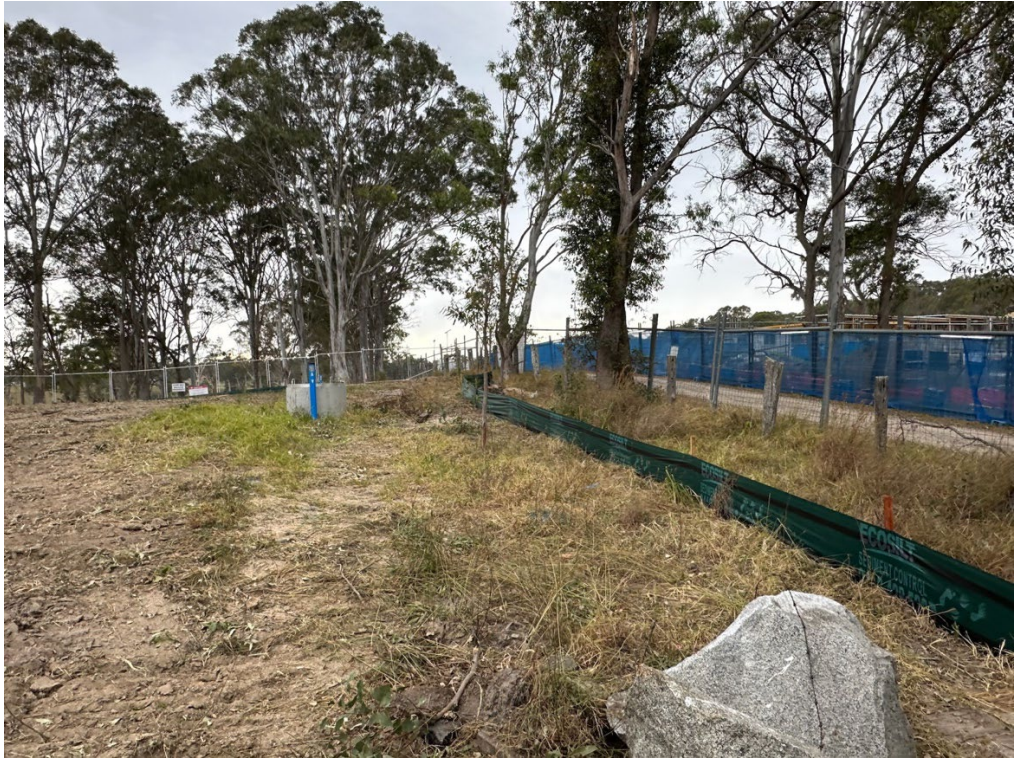
Photo 23: Preparatory works, road tie into Caswell St
