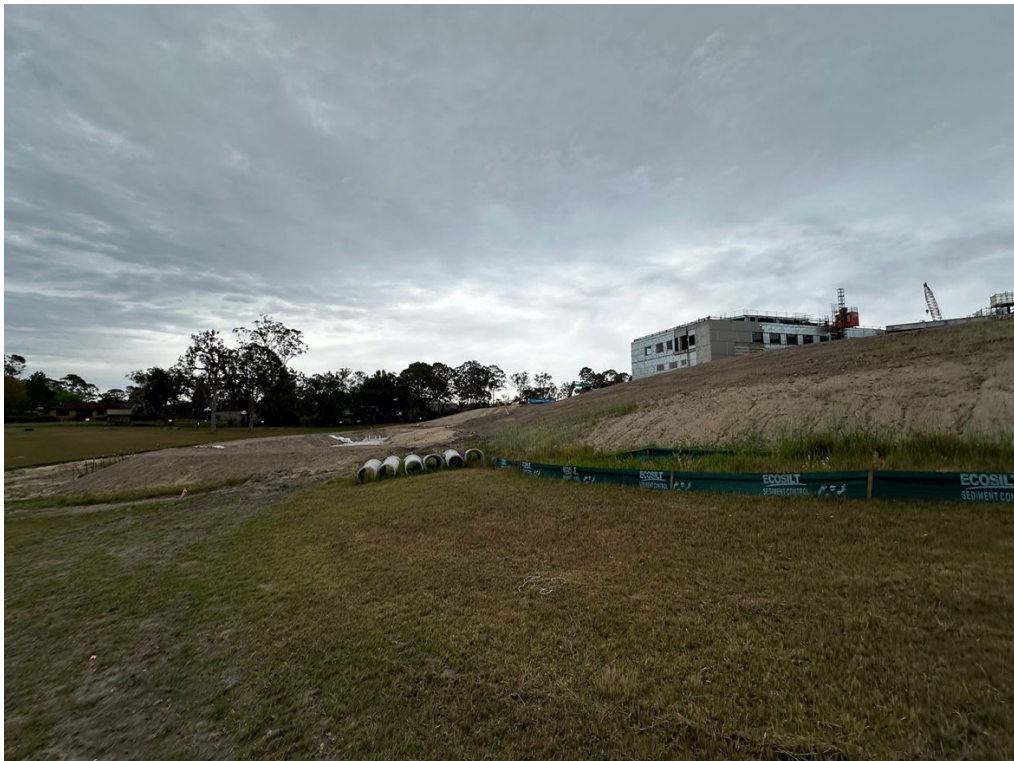
Photo 10: Construction Sediment Basin
