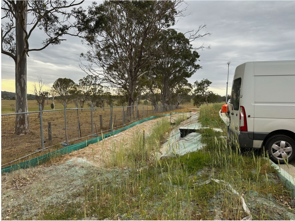
Photo 11: Perimeter drain
