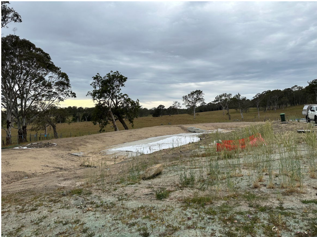
Photo 12: Construction Sediment basin undergoing conversion to operational basin
