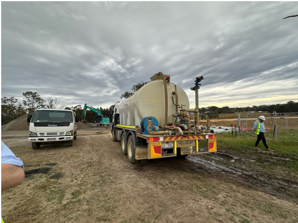
Photo 9: Water tank with jet hose attachment for dust suppression
