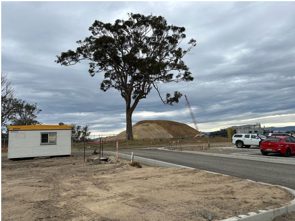
Photo 14: Tree Protection zone and stockpile
