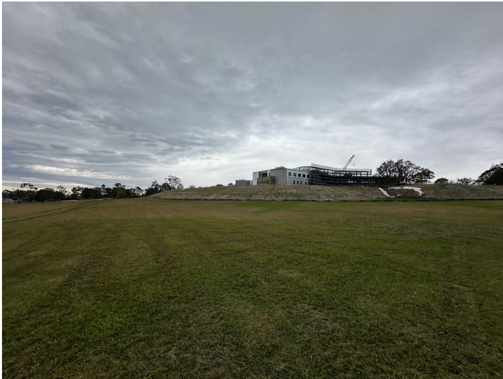
Photo 1: Main Building Construction
