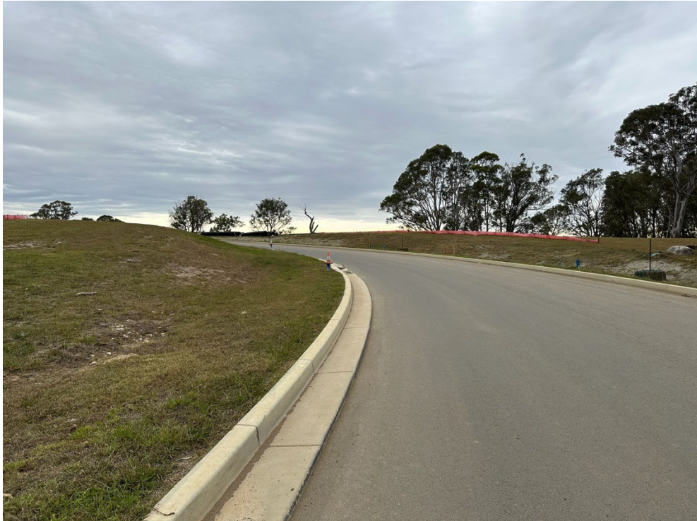
Photo 6: Sealed internal access road and stabilised batter
