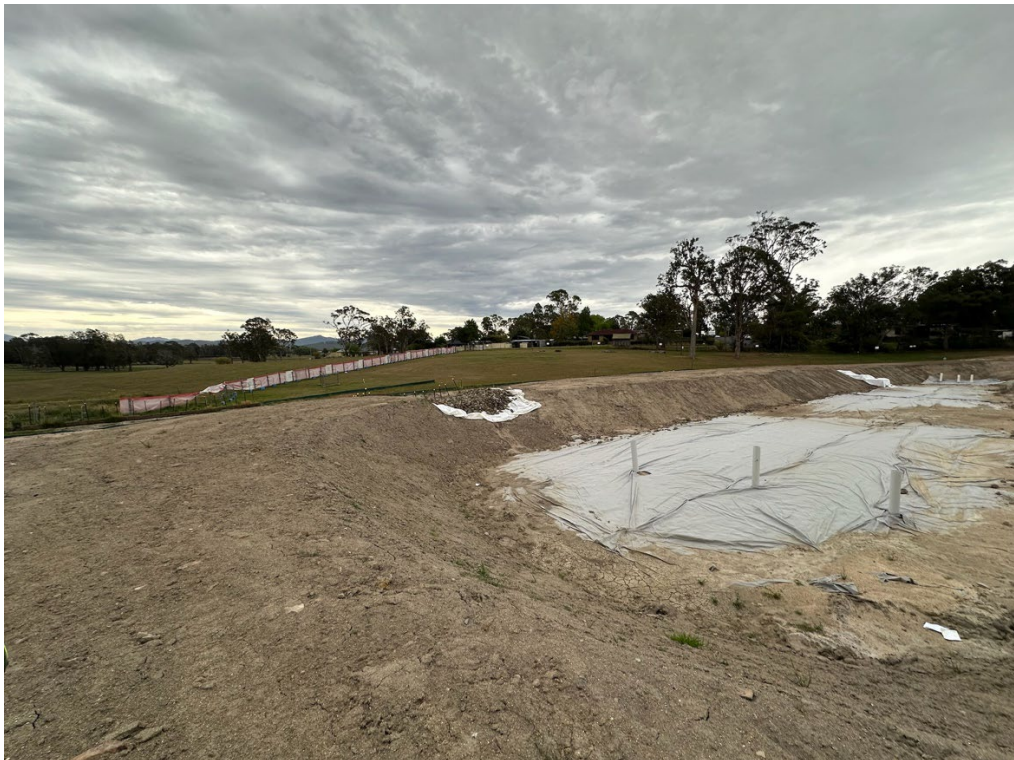
Photo 8: Sediment basin undergoing conversion to operational basin
