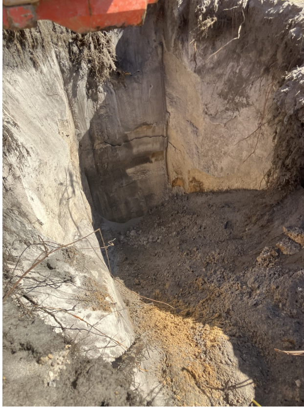
Test Pit - 0.00mbgl to 1.20mbgl
