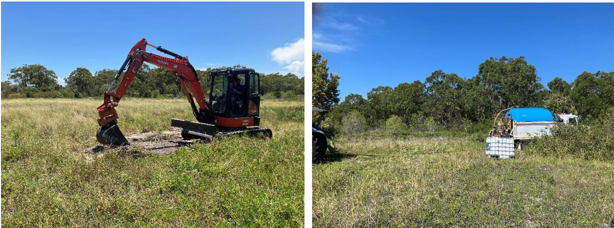
Figure 1-3. Photos of Site 2: Left: Looking east at an excavator preparing to dig TP4. Right: Looking south at the water tanker near TP1.
