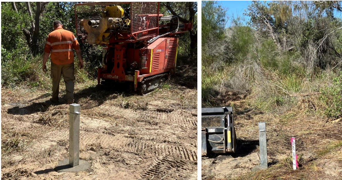
Figure 2-2. Finished piezometer upstands; BH5 to the left and BH7 to the right.
