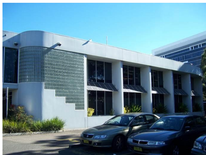
Figure 9. Northern elevation of existing warehouse/office building
