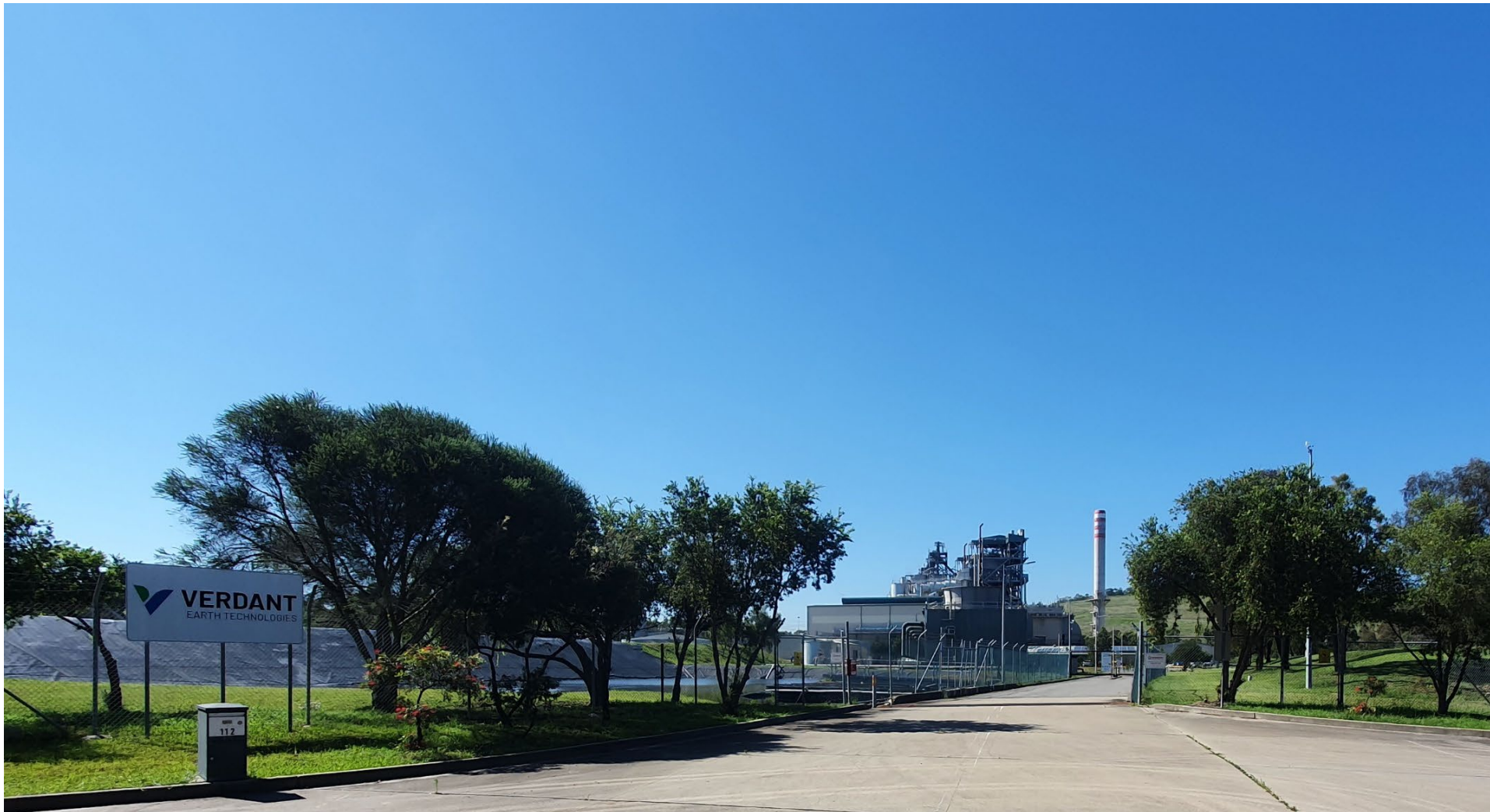
Figure 20.3. View of the front of the Site showing dominant Site features.
