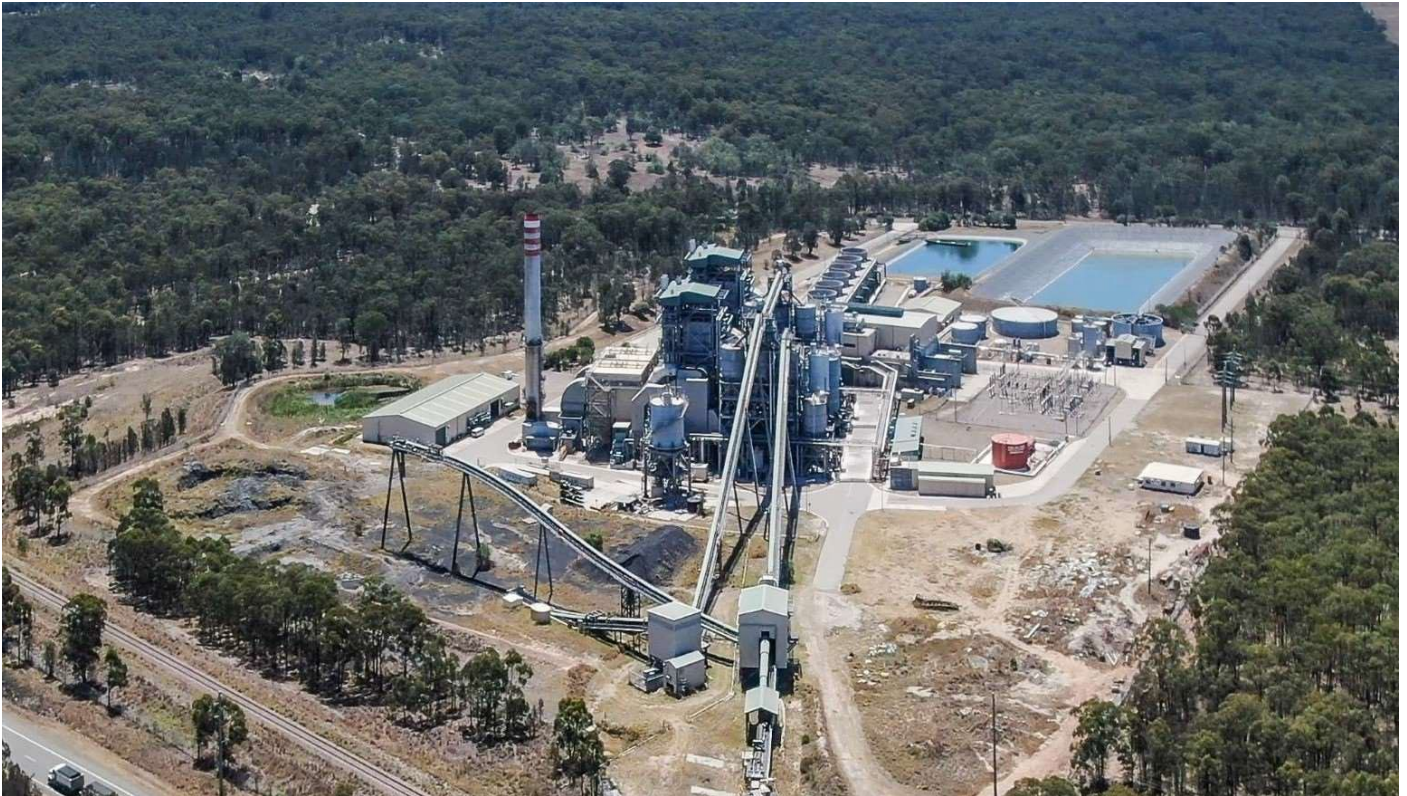
Figure 1.5. View of Redbank Power Station from the south.
