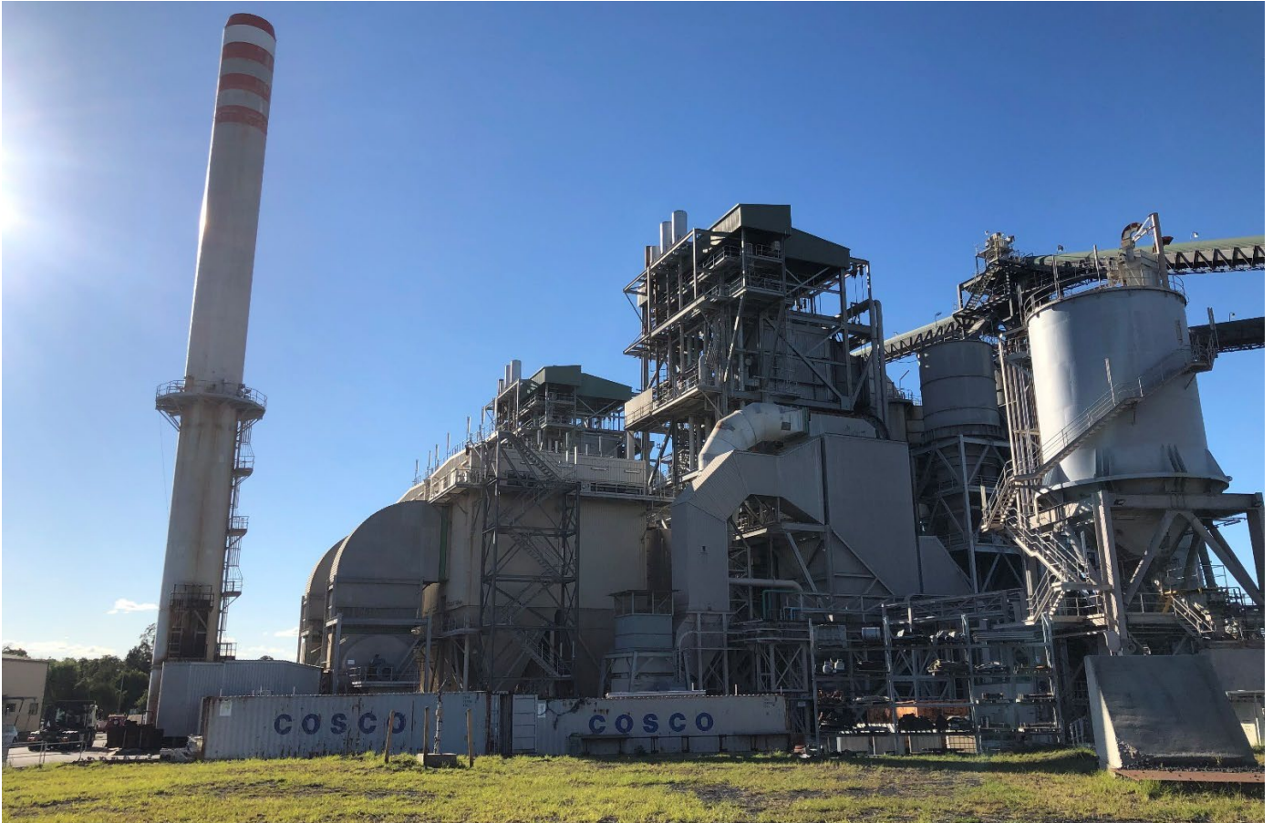
Figure 1.6. View of the south side of the Redbank Power Station.
