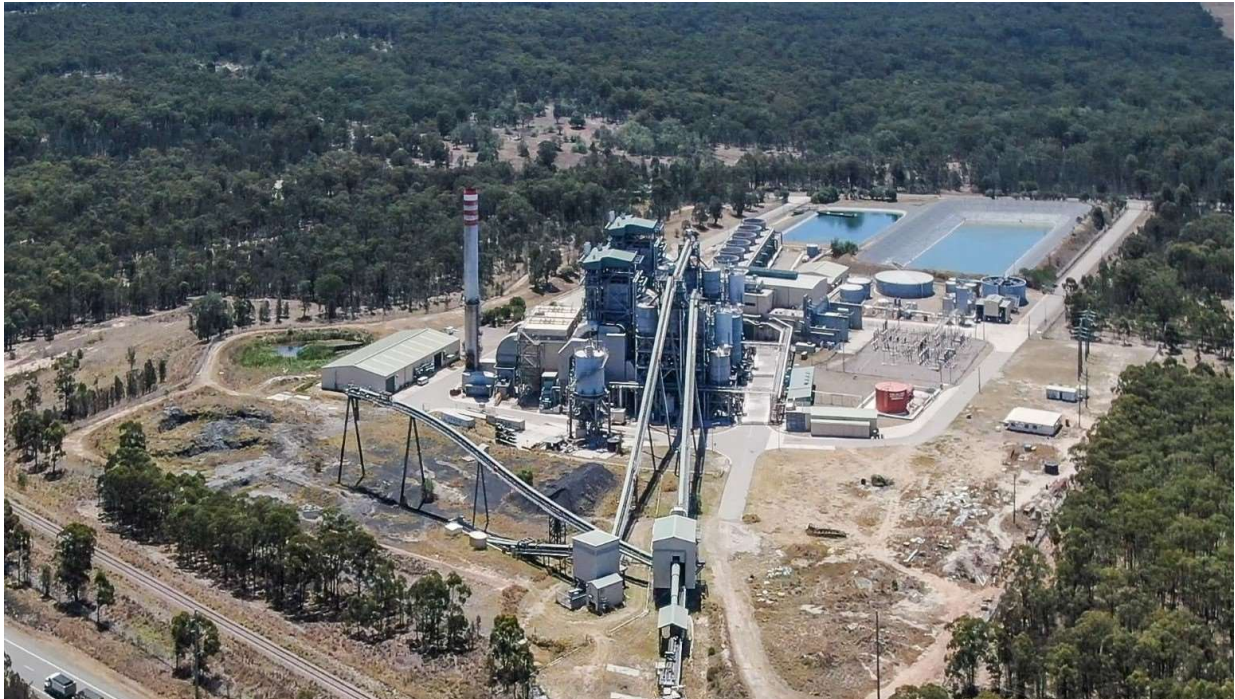
Figure 2 - View of Redbank Site from South
