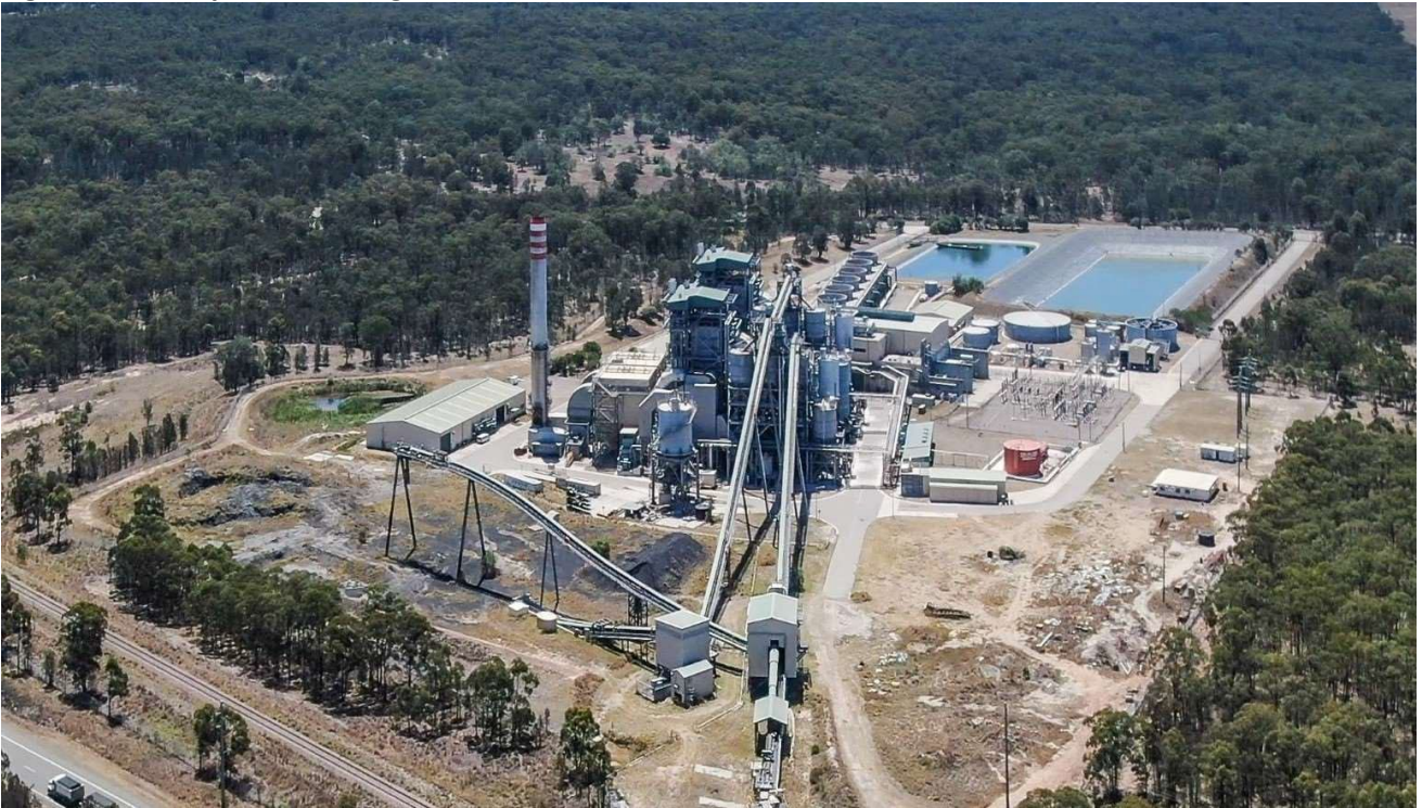
Figure 1.6. Oblique aerial image of Redbank Power Station from the south.
