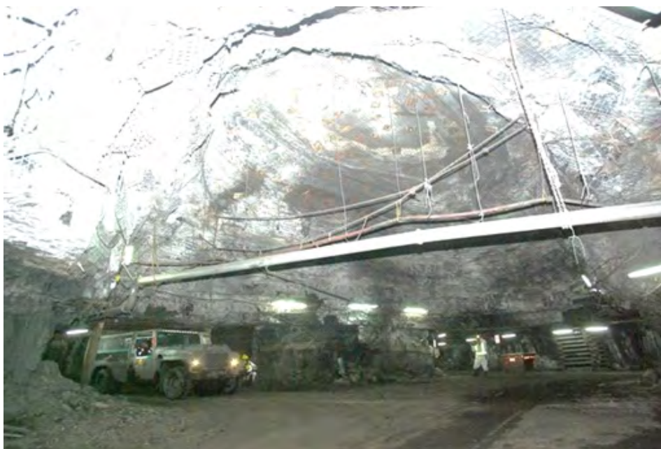
Photograph 8.1: Recovered Roof Fall at Angus Place – approximately 7 m high and 10 m wide
