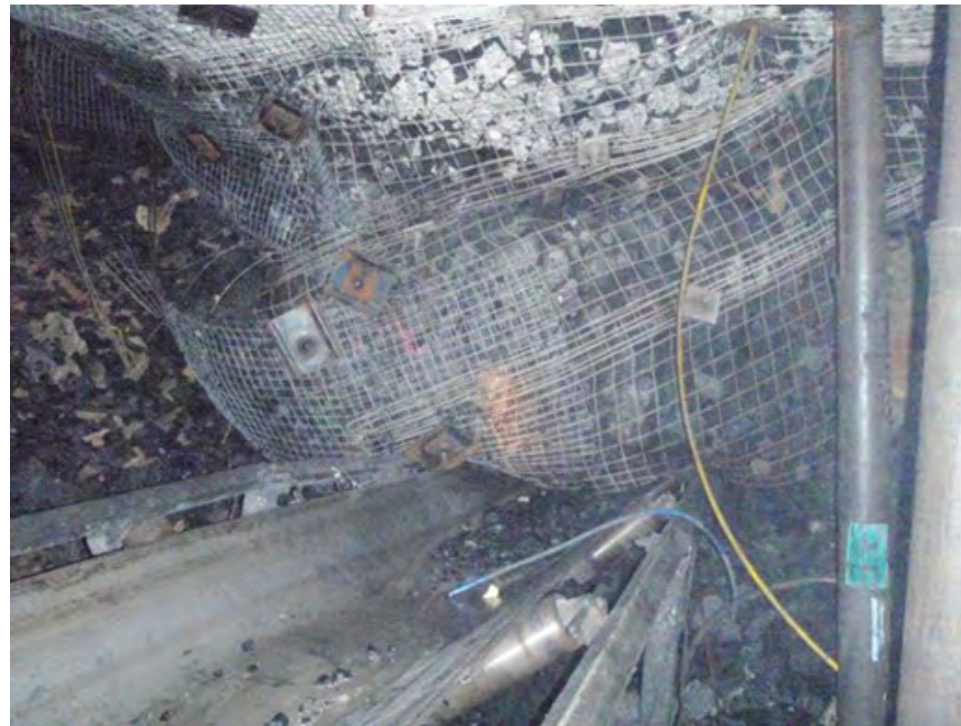
Photograph 8.2: Roof Fall on longwall belt at Springvale – approximately 6 m high and 20 m long
