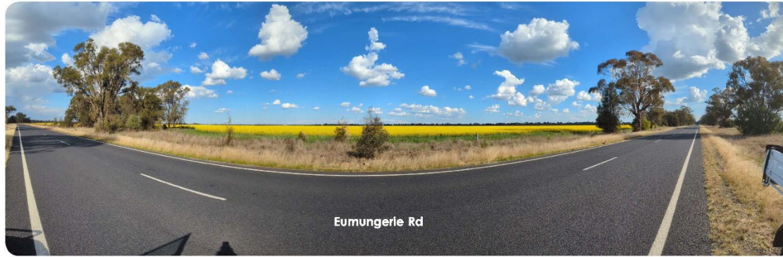
PANORAMA SITE PHOTO provided by Kleinfelder File Name: PXL_20230828_050131283.PANO - View 9
