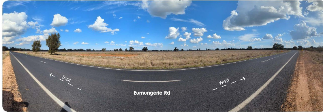
PANORAMA SITE PHOTO provided by Kleinfelder File Name: PXL_20230828_045749428.PANO - View 4
