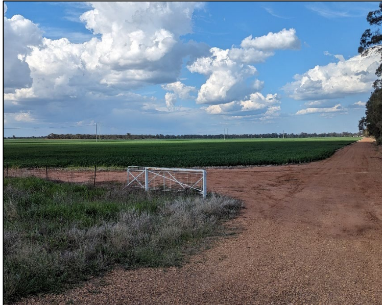
Plate 3-1: Dubbo-Nevertire Essential Energy 132kV Line in Subject Lot Southern Portion
