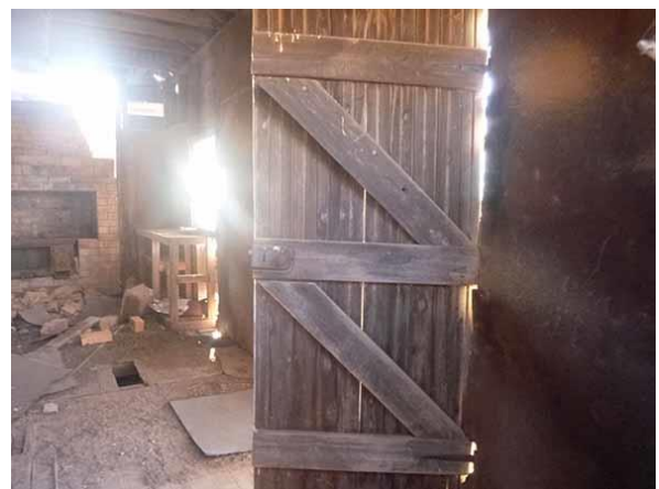
10. Hardwood timber flooring and door.
