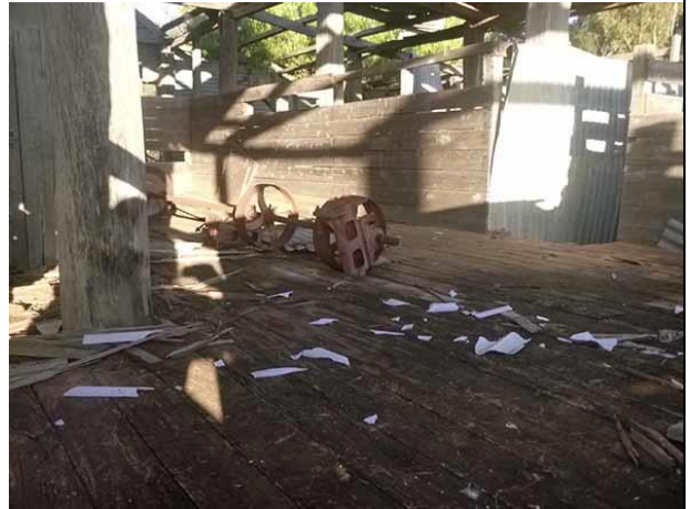
6. Shaft driven shearing equipment. Timber floorboards and internal timber cladding evident
