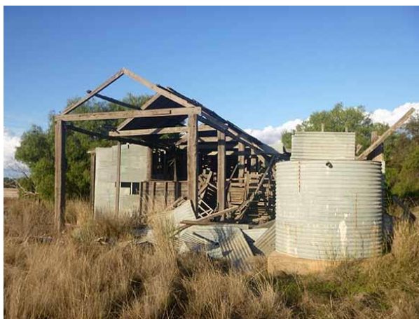
3. Corrugated iron water tank on the southern side of structure
