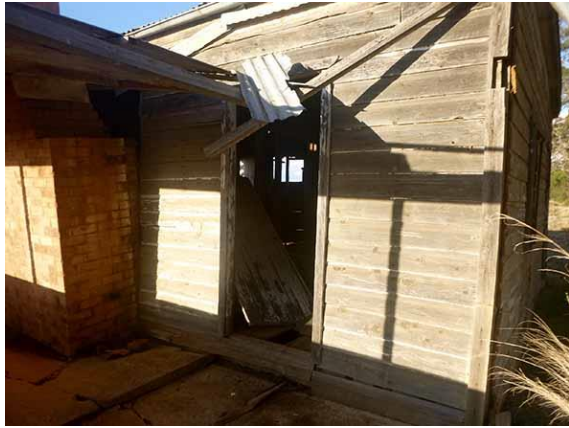
5. Timber cladding along the western side wall.
