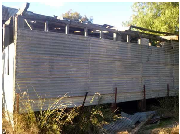
8. Corrugated iron annex on the eastern side of main structure
