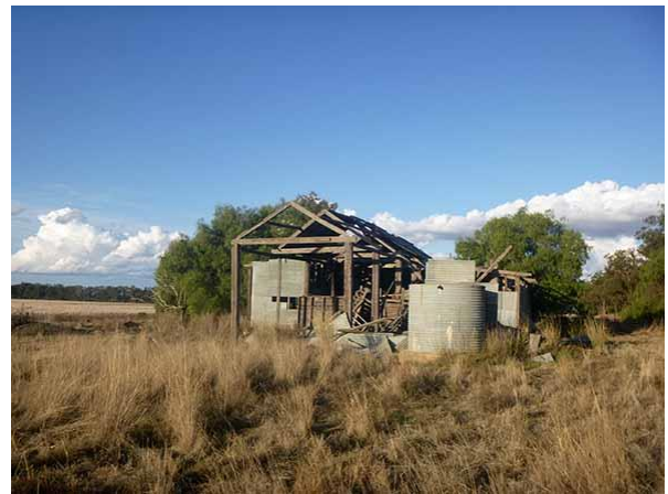
2. Southern end of shearing shed showing exposed timber framing
