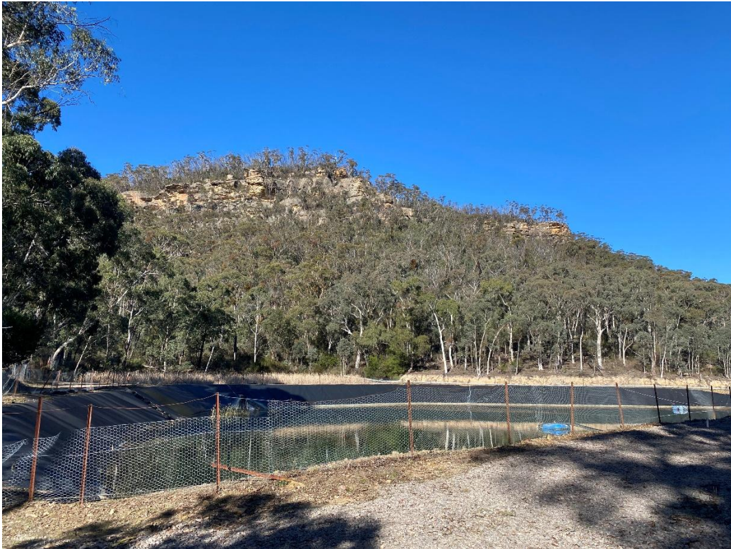
Photograph 23 – Looking up towards main dam
