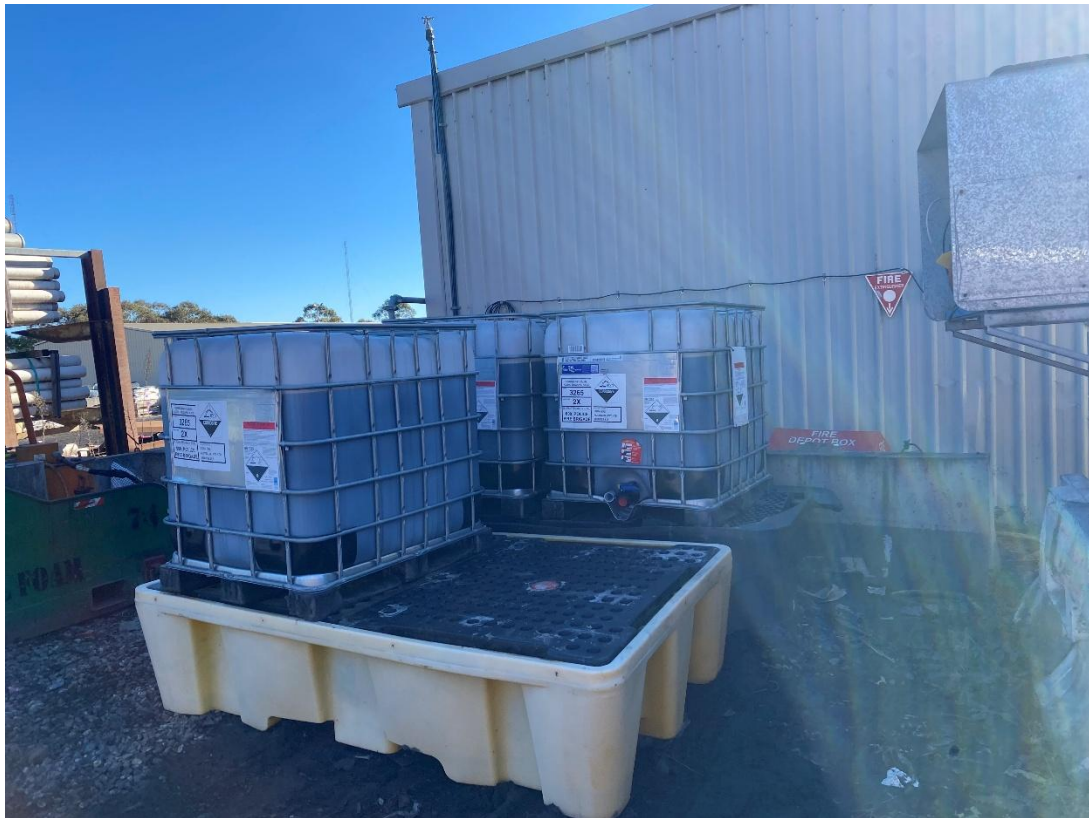
Photograph 29 – Hydrocarbons stored as per AS1940
