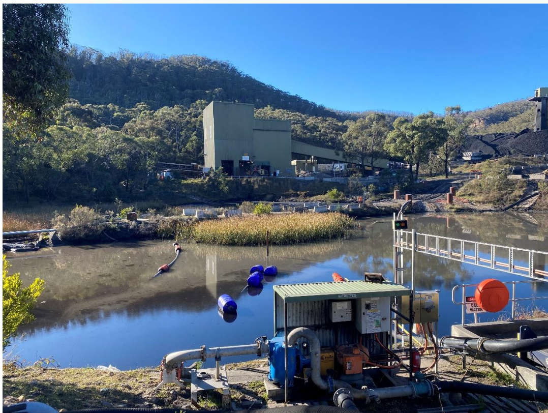
Photograph 38 – Coal stockpile pond and looking back to stockpile area
