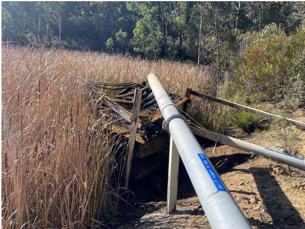
Photograph 24 – Flow control structure
