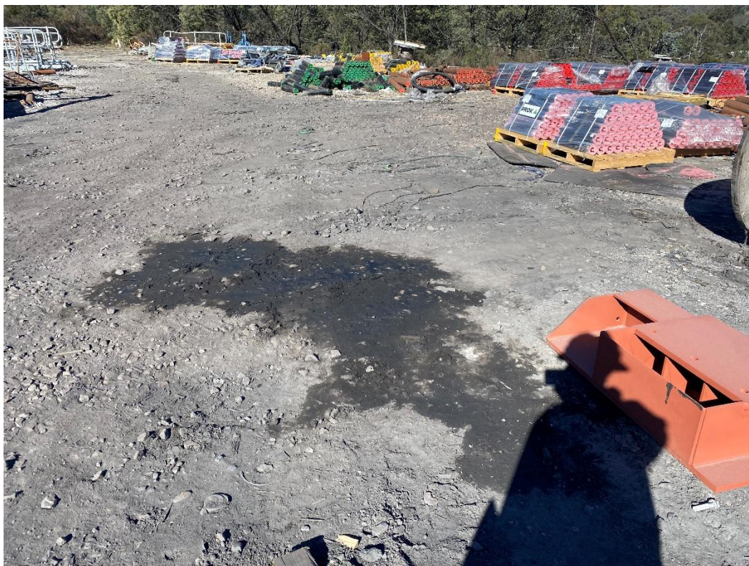
Photograph 13 – Hydrocarbon staining in laydown area
