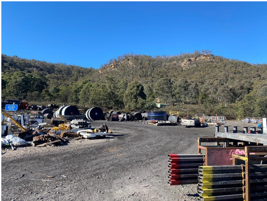
Photograph 10 – Example of laydown area
