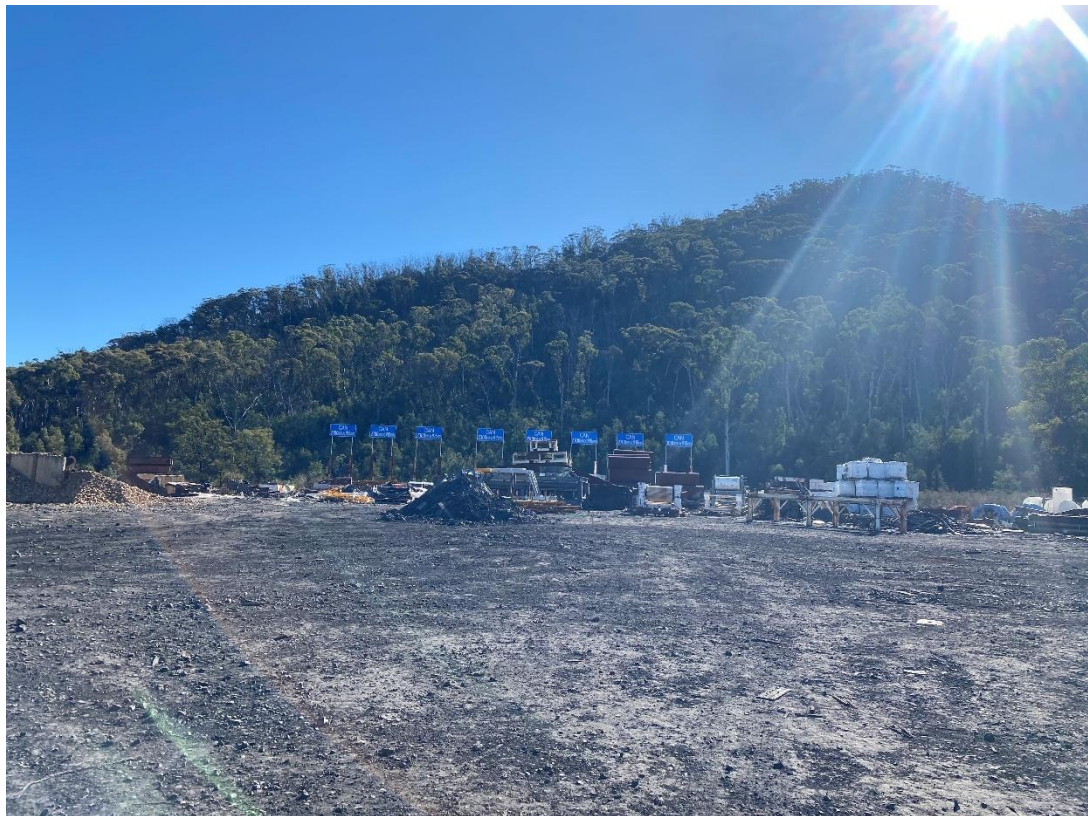
Photograph 18 – Segregated waste area
