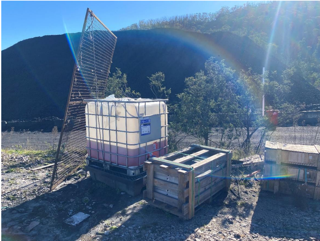
Photograph 11 – 1000L IBC containing hydrocarbons not stored as per AS1940
