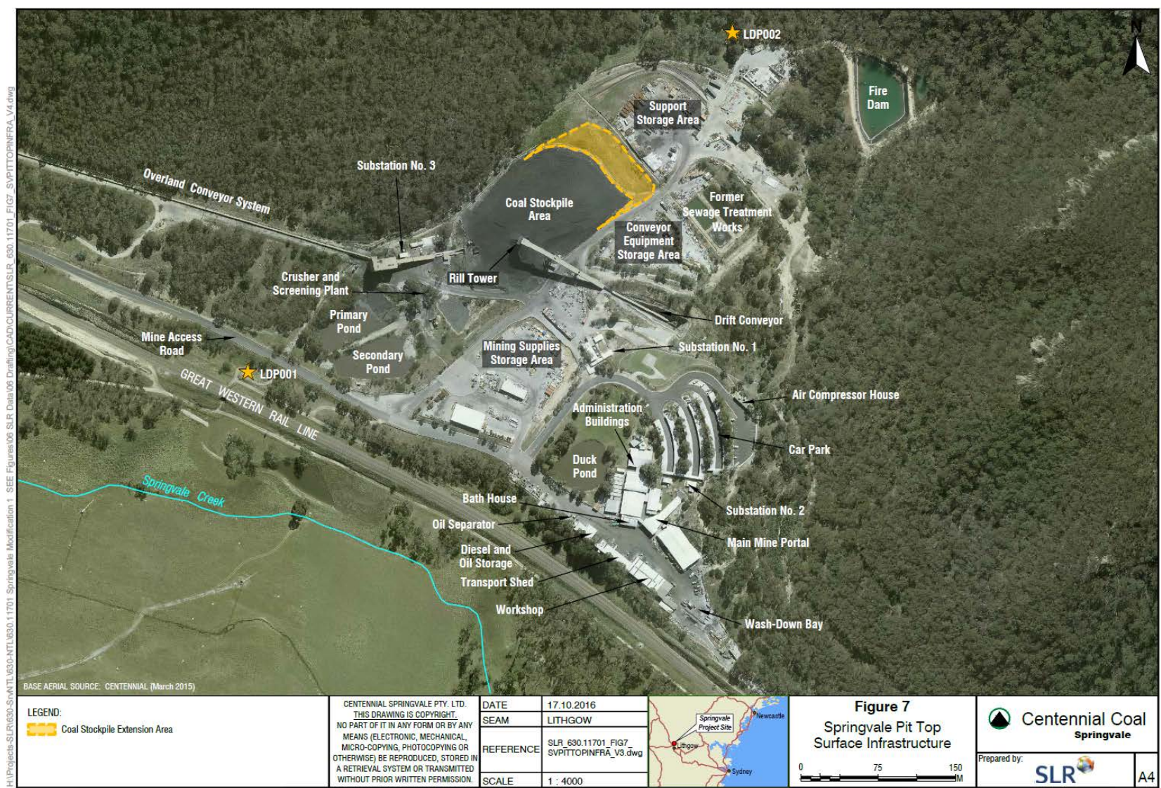
Pit Top Surface Facility
