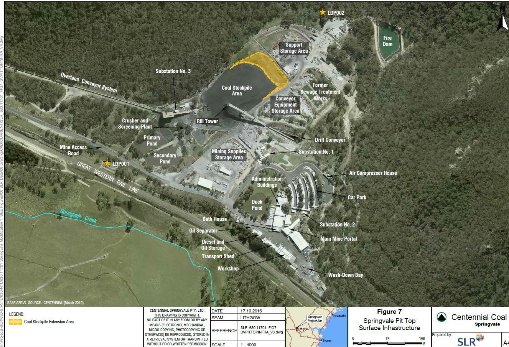
Pit Top Surface Facility
