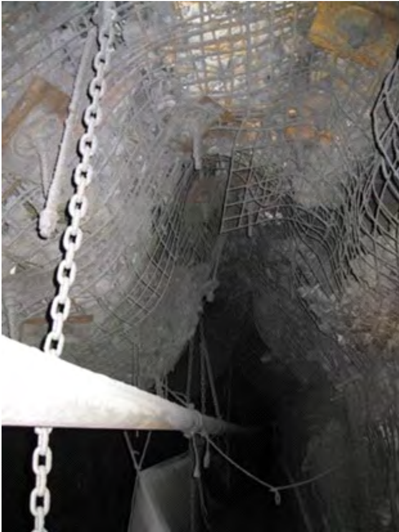
Photograph 8.2: Roof "Guttering" at Angus Place – normal roof horizon is at the level of the pipes
