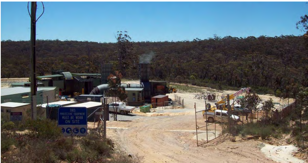
Plate 15: Air Vent Shaft
