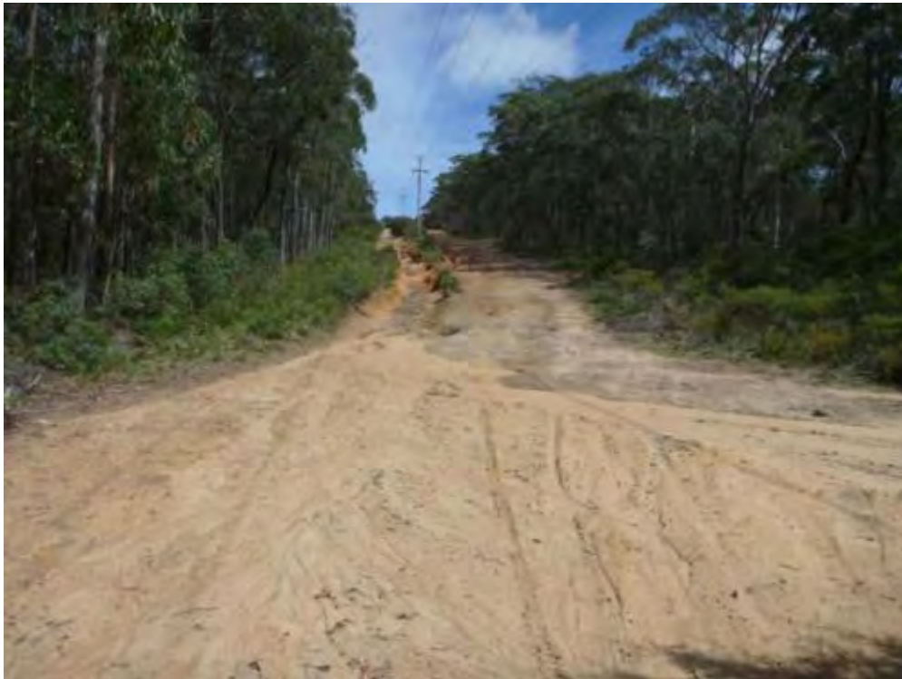
Plate 21 Survey unit 13 – powerline easement.
