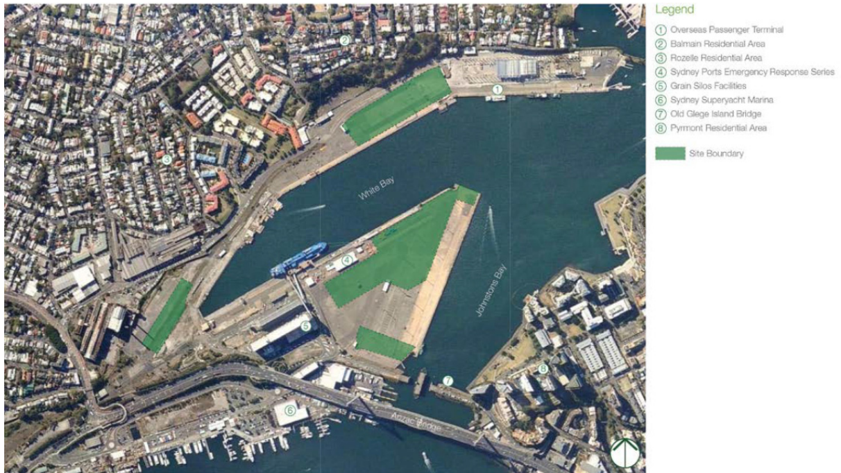
Figure 2: Location of the development across Glebe Island and White Bay shown in green (source: Environmental Impact Statement, Glebe Island Expo, AAP, November 2012, page 14).
