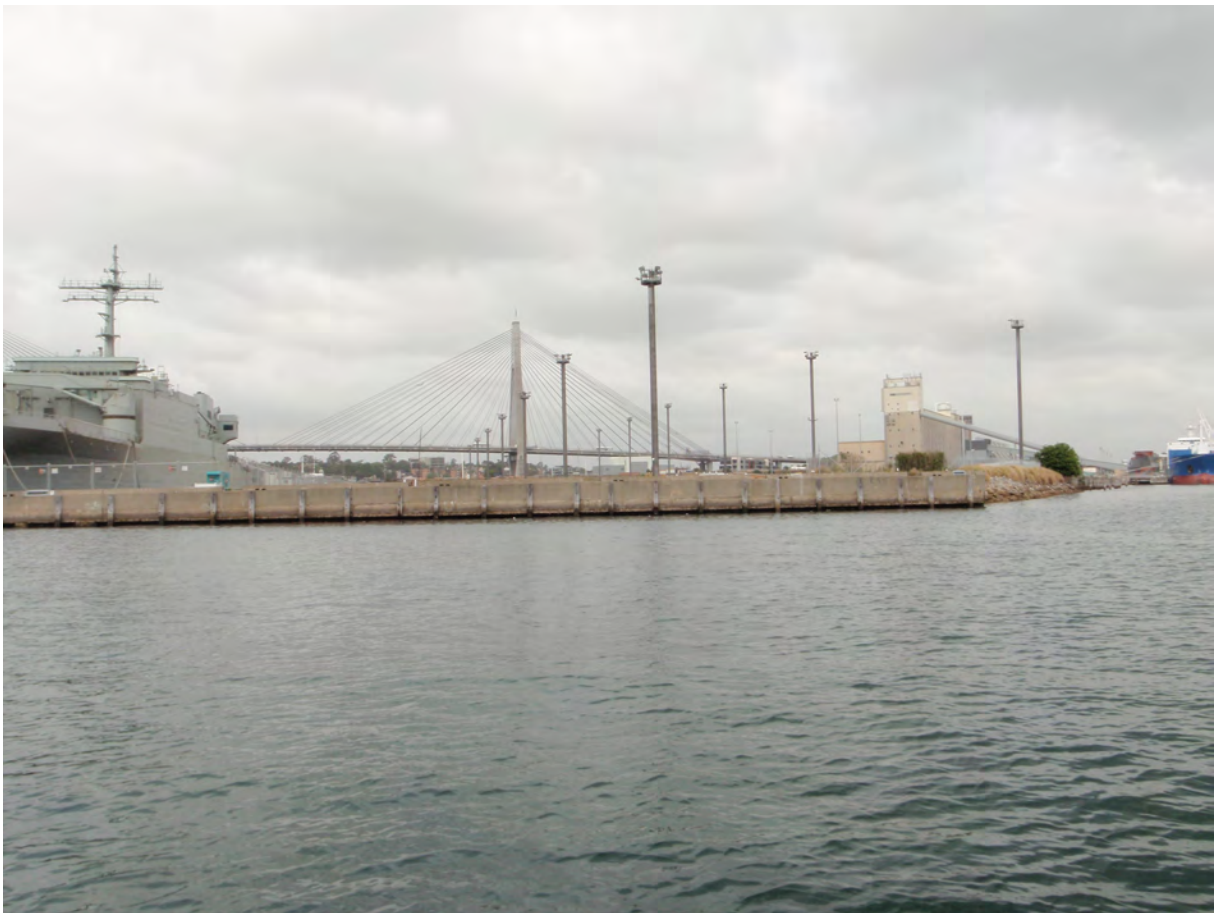
Figure 1 View of Berth 3 at the northern end of the Glebe Island Terminal, Johnson Bay.
