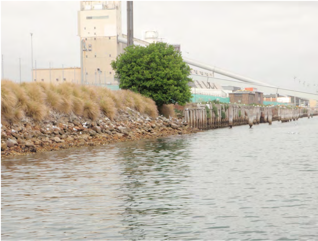
Figure 5 View of rip-rap revetment wall looking south towards the disused Berth 5 piles. The Cement and Sugar Terminals are located further south at Berths 6 and 7.
