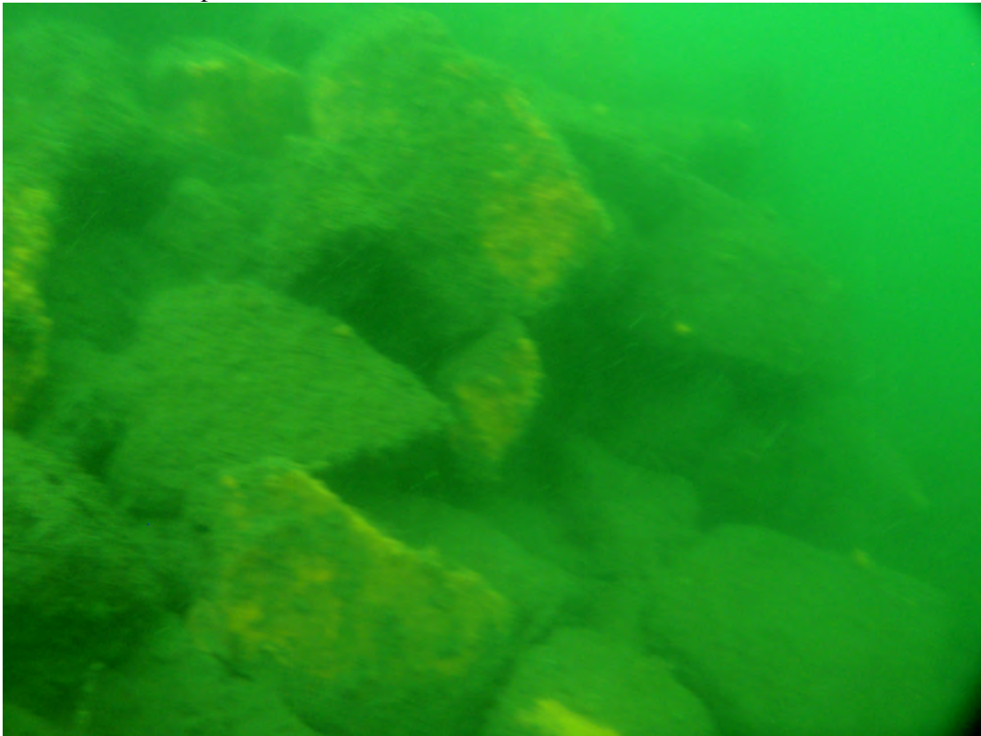
Figure 21. Silt smothers most encrusting growth and aquatic plants on the revetment rocks from about 3m depth down.
