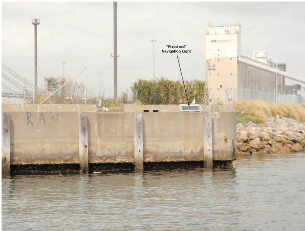
Figure 25 North-west side of Glebe Island berth 3 showing north facing “fixed red” navigation light. There is a similar light on the west facing side and two others at the north-eastern and east sides of the berth.
