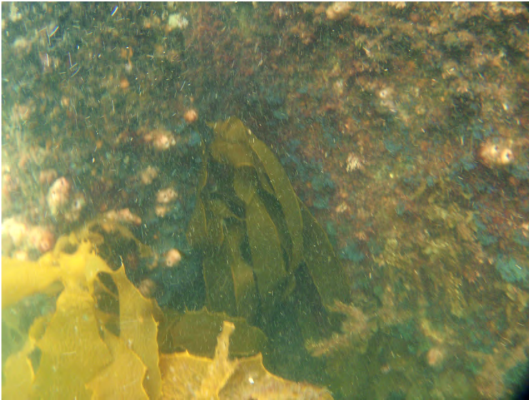
Figure 15 Mixed kelp, frondose algae and tunicate zone in deeper sub-tidal below subtidal fringe on concrete wall.
