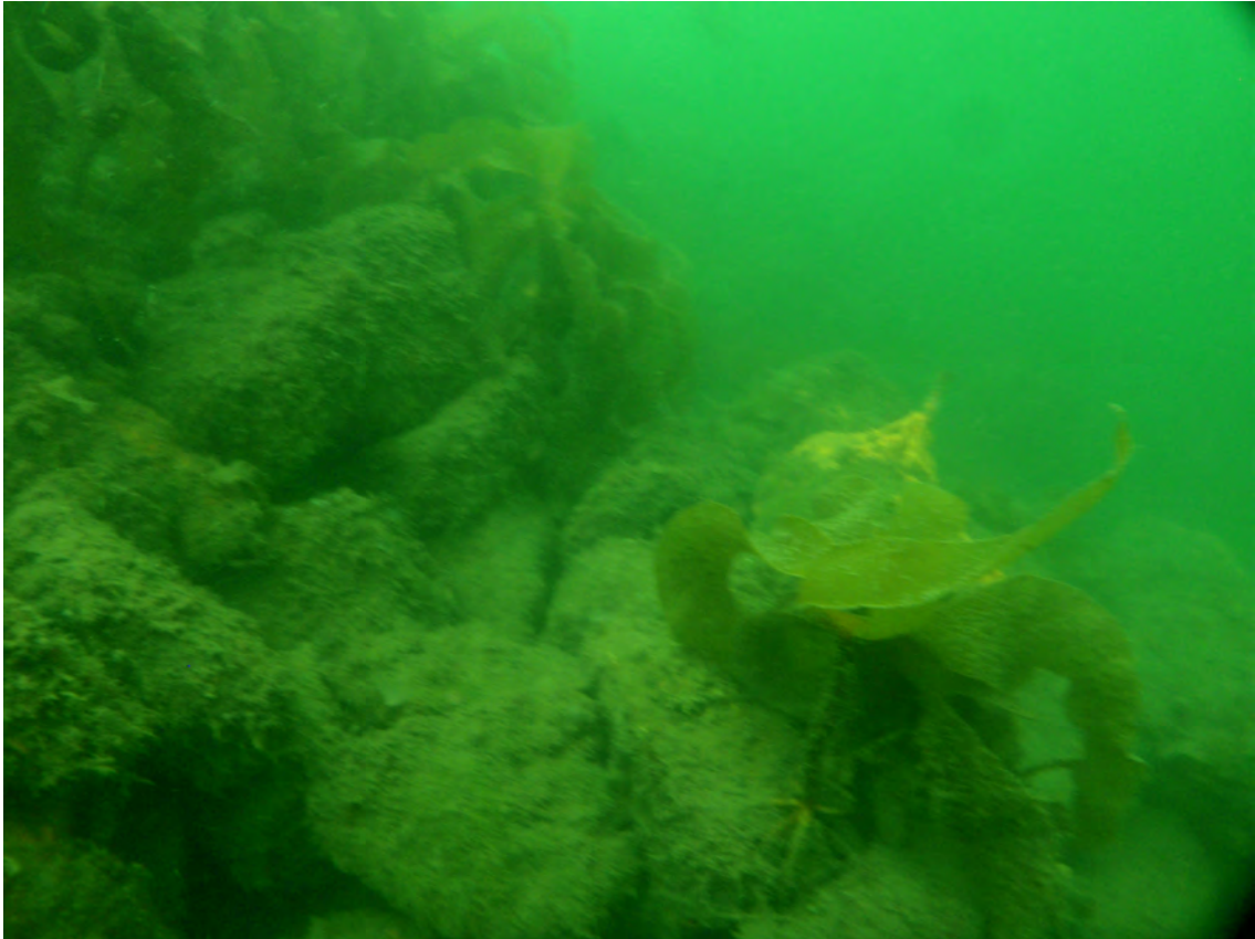
Figure 21. Silt smothers most encrusting growth and aquatic plants on the revetment rocks from about 3m depth down.
