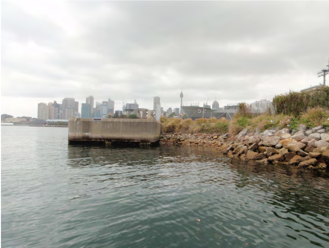
Figure 4 View of western side of Berth 3 looking east from off-shore of the rip-rap revetment (unused Berth 4).
