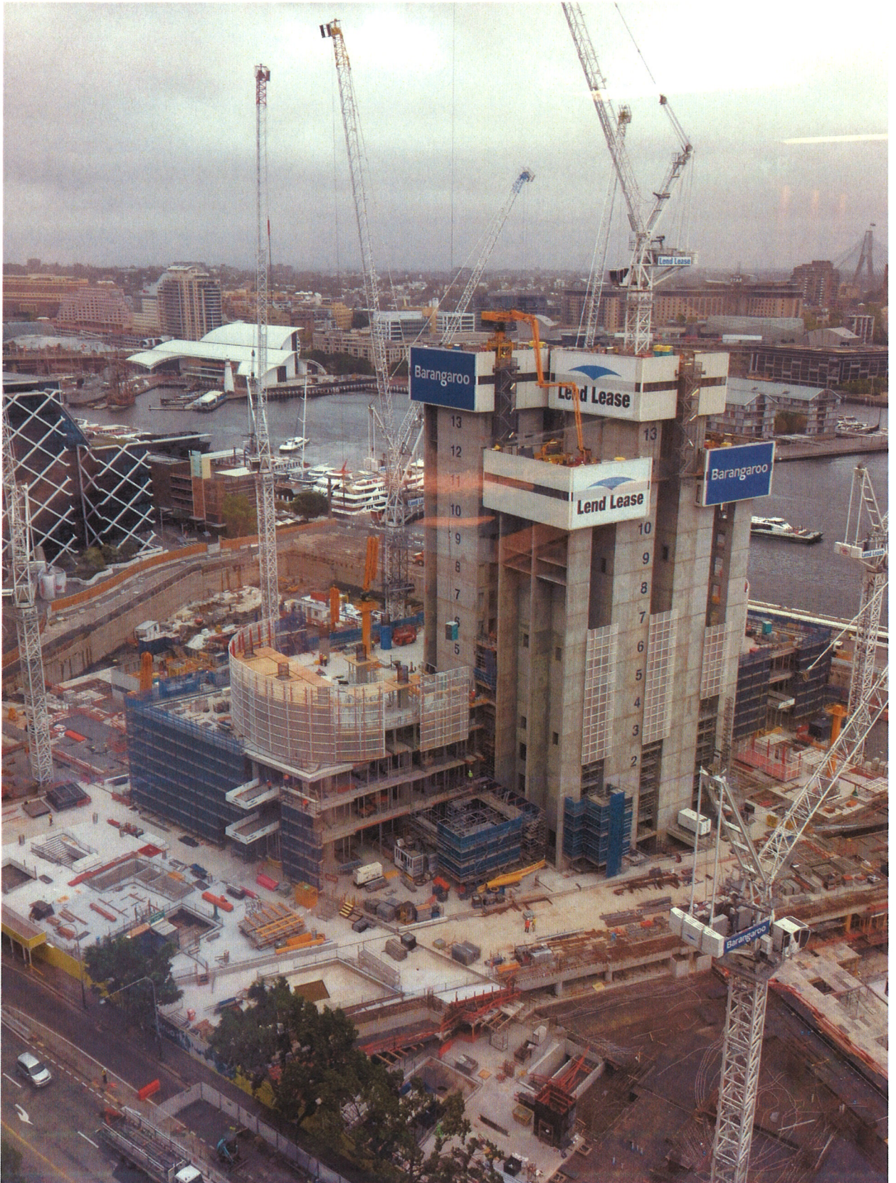
Figure 2: Construction of Commercial Building C4 (photo taken 4 February 2014)
