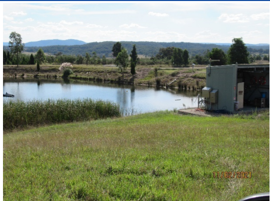
Photo 18 Discharge Dam/Production Dam with adequate freeboard and presence of reeds in dam. Water is re-used back into the mining operation from this dam and pump house. (SSD_5581 Schedule 4 Condition 10 and EPL12374 Condition O4.1).
