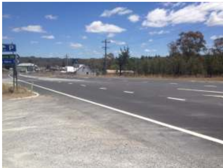
Plate 2 - Castlereagh Highway / Glen Davis Road Intersection
