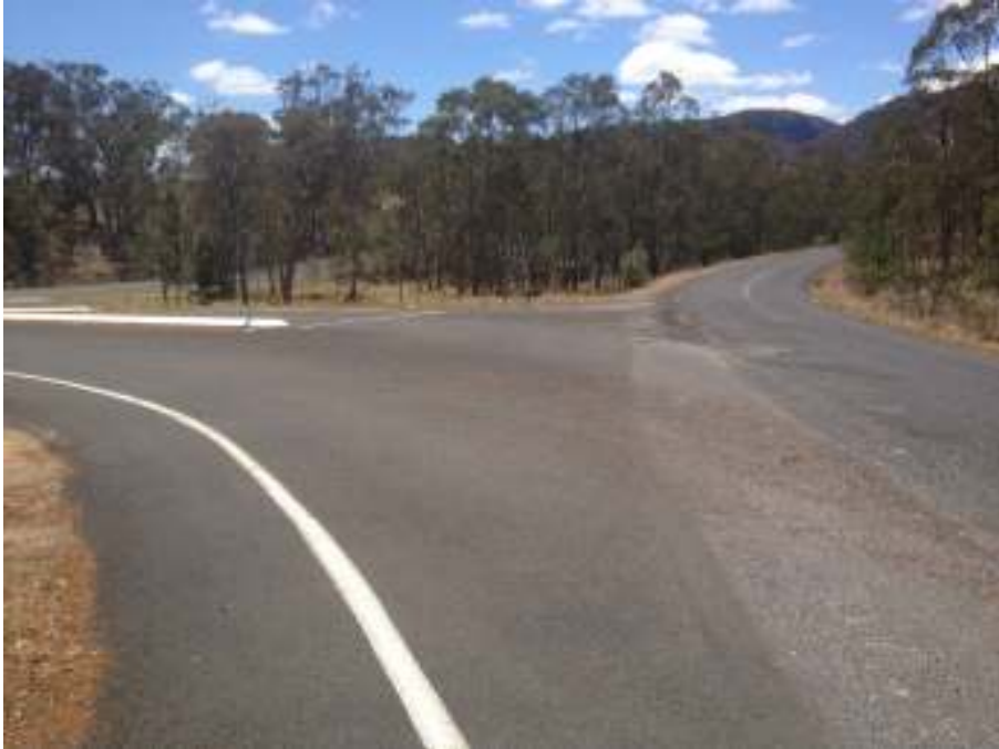
Plate 3 – Intersection between Glen Davis Road and Mine Access Road
