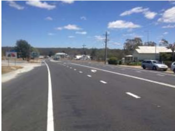
Plate 1 - Castlereagh Highway / Glen Davis Road Intersection
