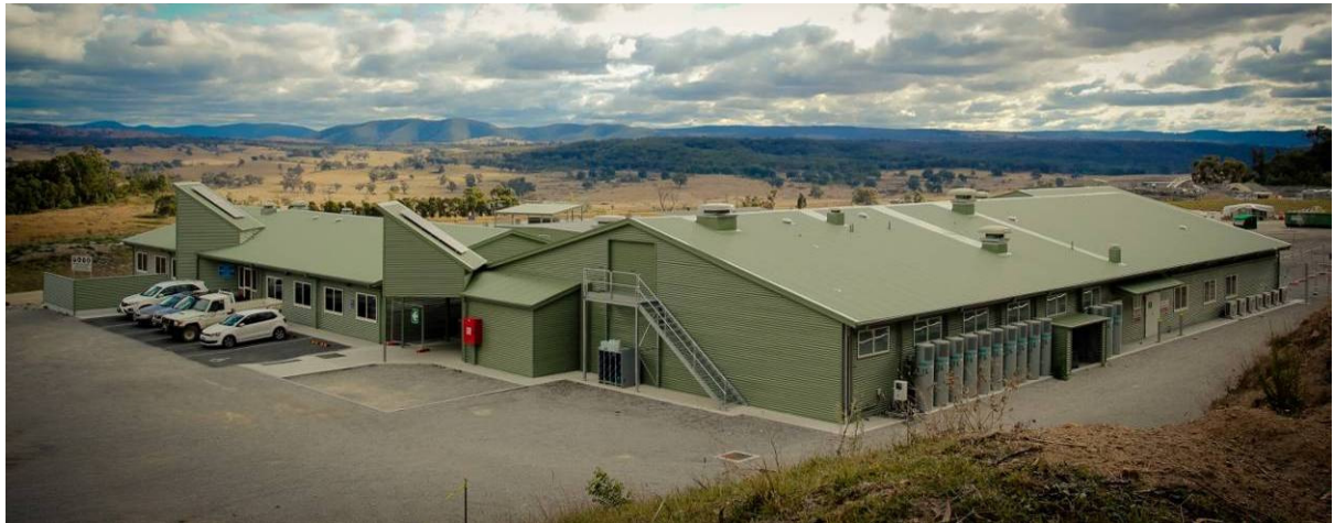
Plate 1: Airly Administration Building
