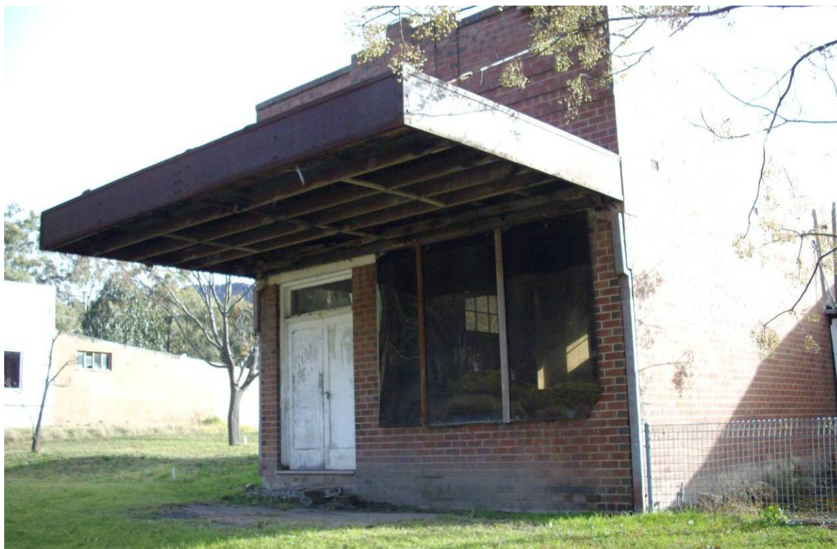
Plate 11: Disused Shop at Glen Davis
