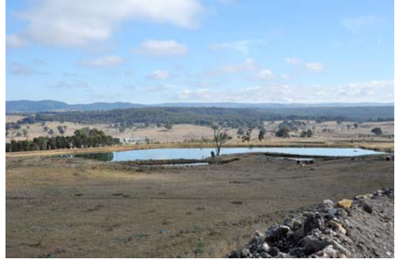
Plate 8 Sediment Control dams
