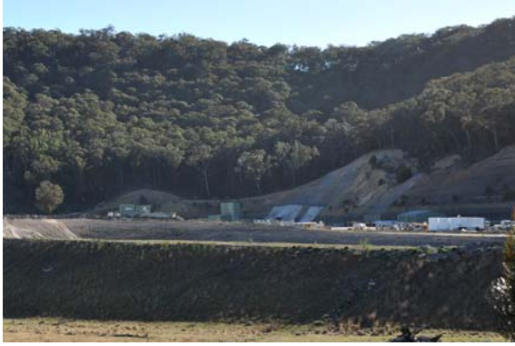
Plate 7 Ventilation and mine access portals
