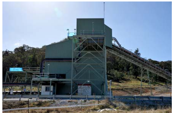
Plate 4 Coal crusher and screening plant
