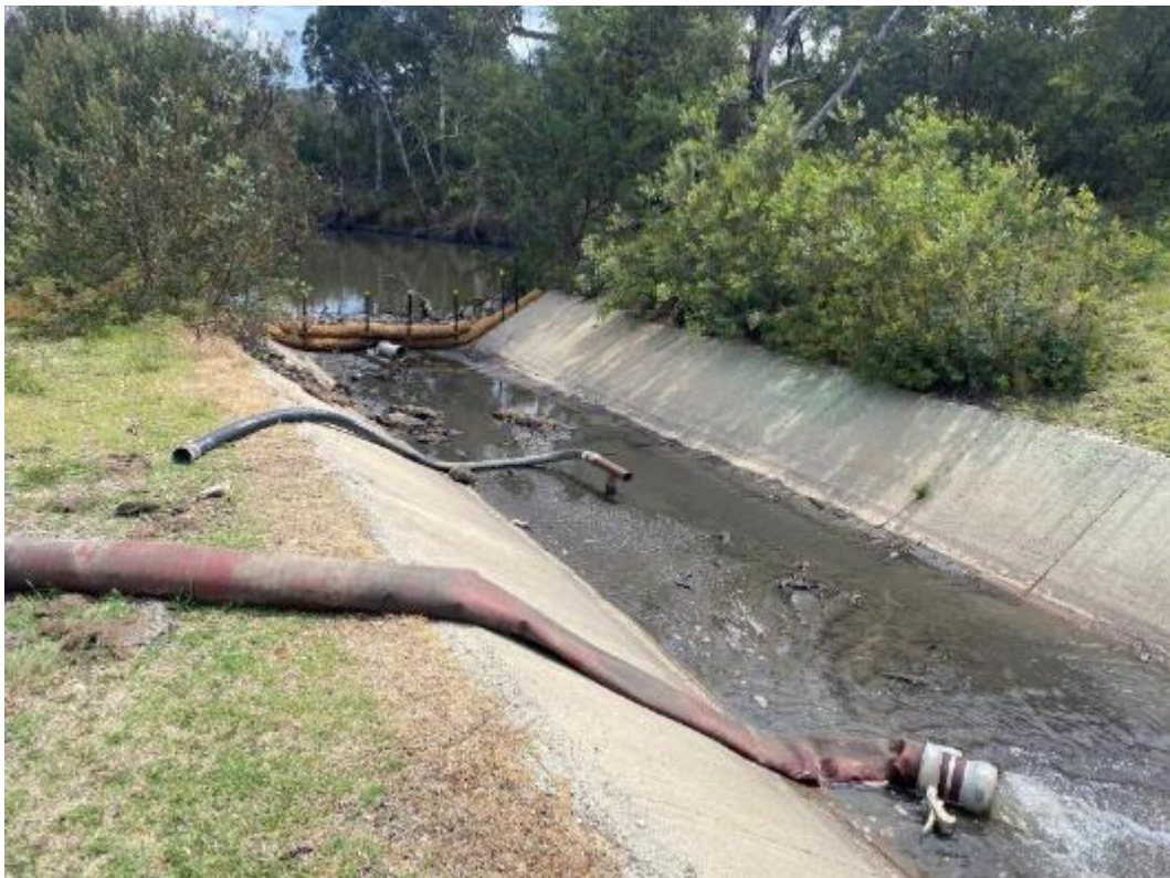
Photo 06 - Dam and Drain at Springvale Coal Services
