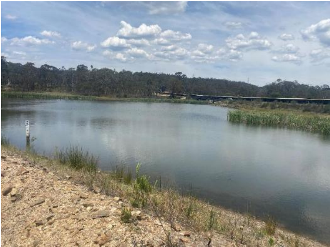
Photo 04 - Main Dam at SCSS
