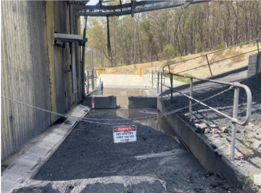
Photo 01 - Sumps Need Regular Removal
