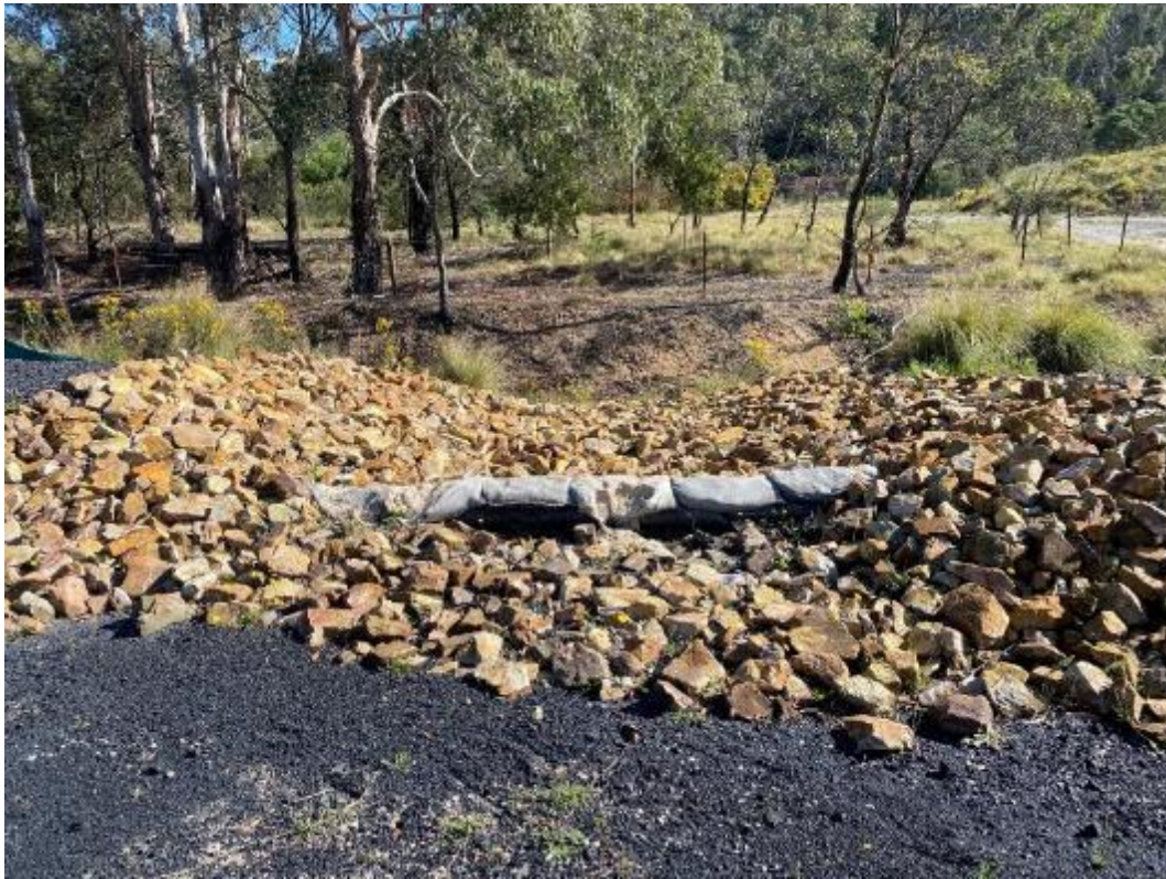
Photo 17 - Effective Erosion Sediment Control at Kerosene Vale
