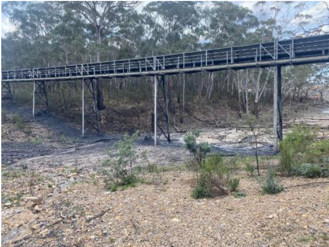
Photo 10 - Carbonaceous Material Can Run into EA Land
