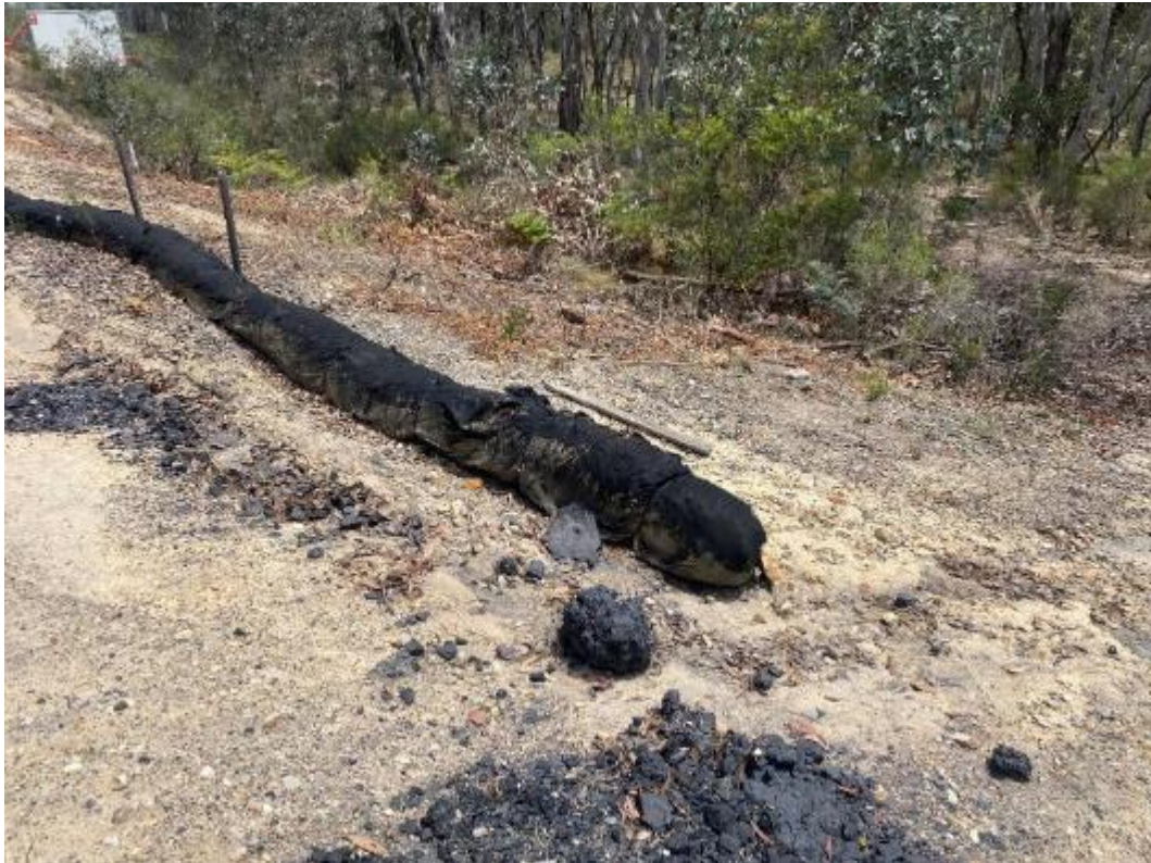
Photo 13 - Coir Logs to be Extended for Erosion Sediment Control
