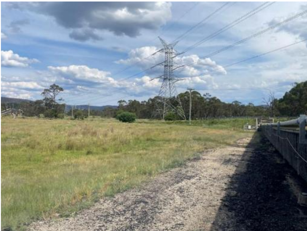
Photo 22 - The LDP Is at a Higher Location Than Where It Discharges at LDP002. See Sign for Low Point
