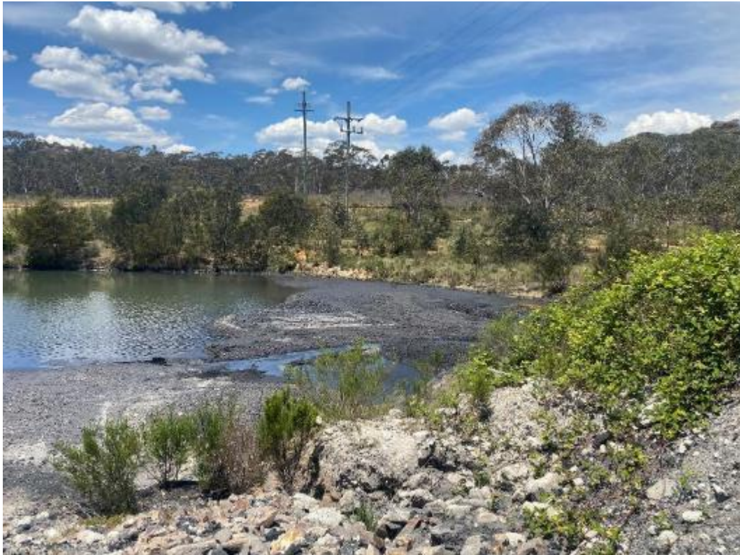
Photo 03 - Desilting is Required in the CHPP Dam
