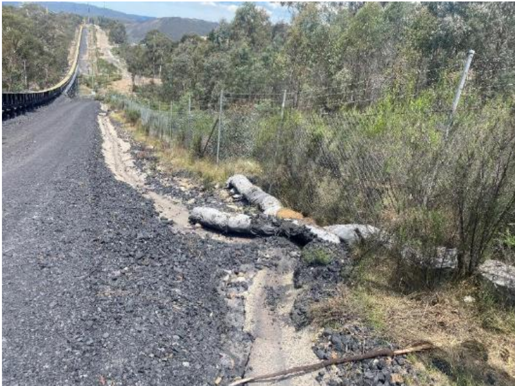
Photo 14 - Temporary Erosion Sediment Control Measures are in Place
