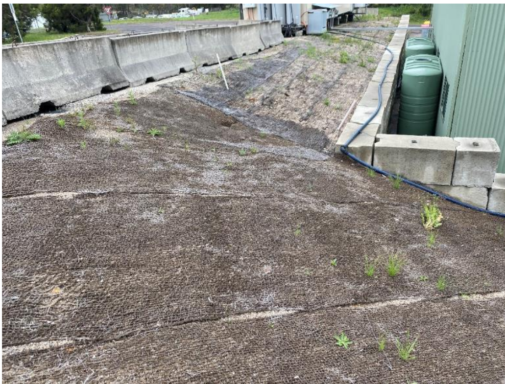
Photo 40: Area to be hydromulched again at Western Coal Services Pit Top (refer IMP REC 13).
