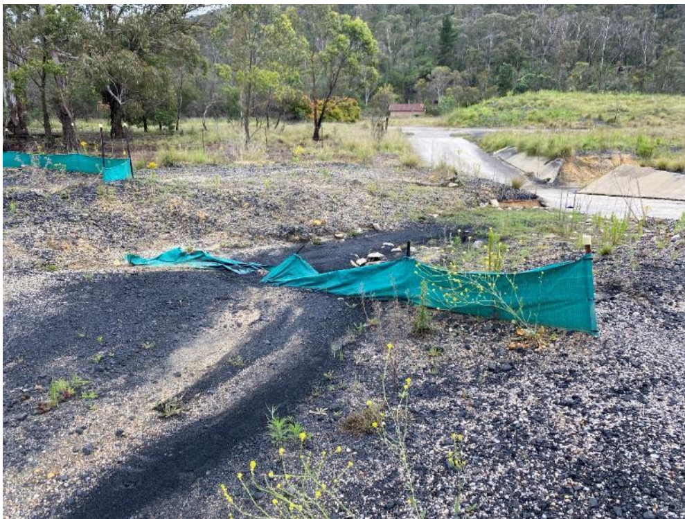
Photo 28: Kerosene Vale – Consider the use of rock structure and/or coir logs in area of failed sediment fence (refer IMP REC 10).
