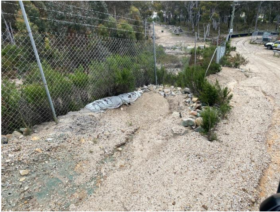
Photo 7: Rock drains near the boundary of Energy Australia and Centennial require clean out (refer IMP REC 5).
