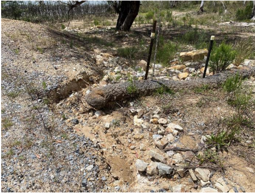
Photo 5: Repair required at 50m of drainage line prior to Main Sediment Dam. Install new coir log (refer IMP REC 4).
