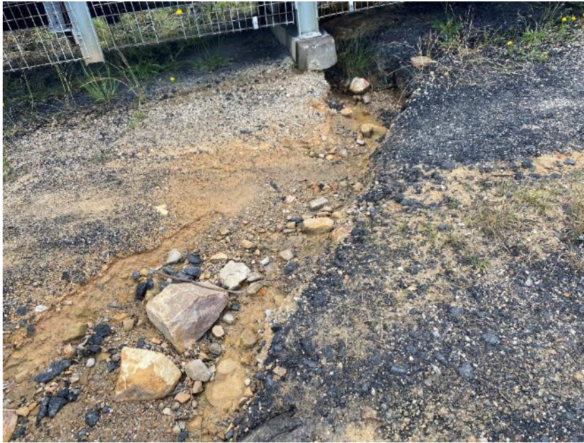
Photo 1: Minor areas requiring erosion repair along conveyor route (refer IMP REC 3)
