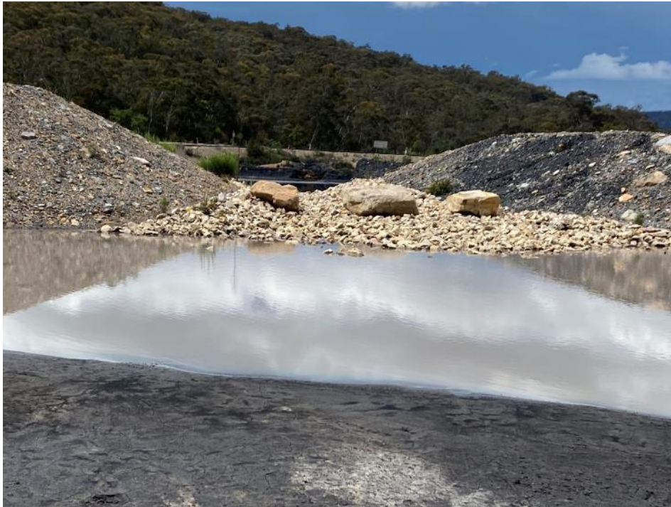
Photo 17: Water build up in area above A Pit. Needs engineering review to confirm integrity and identify solutions (refer IMP REC 6).
