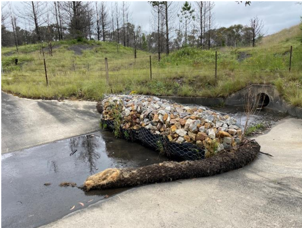
Photo 38: Coir log to be moved back into place at LDP003 (refer IMP REC 12).
