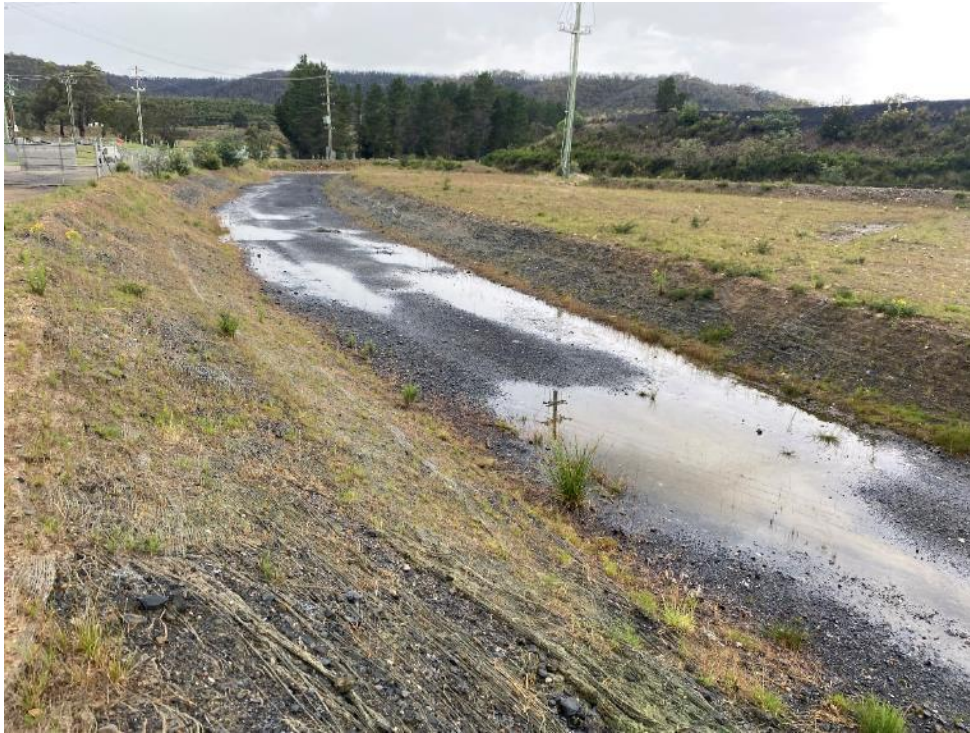
Photo 25: Remove coal in dirty water drain adjacent to main haul road and clean water drain (refer IMP REC 8).
