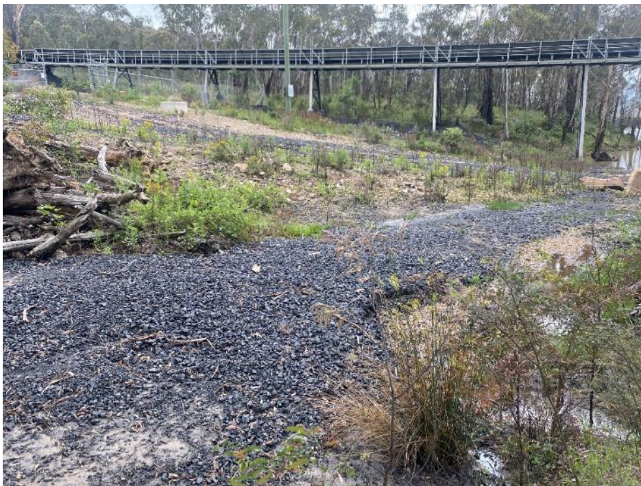
Photo 10: Area at the base of the large hill has a large deposition of coal material with requires removal (refer IMP REC 16).
