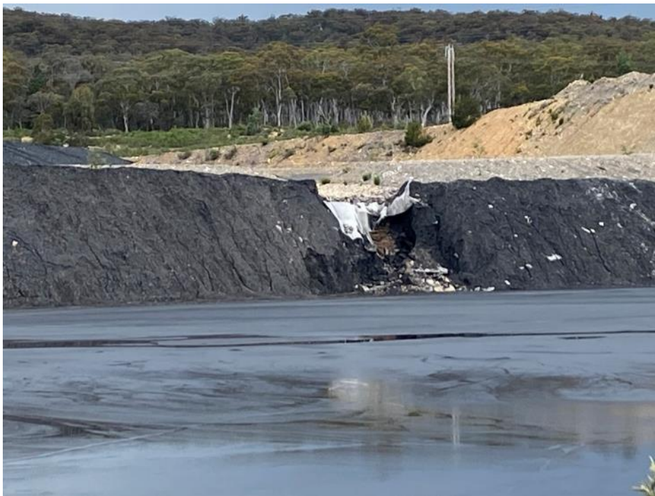
Photo 16: Weak point in the wall of A Pit from water running into A Pit (refer IMP REC 6).
