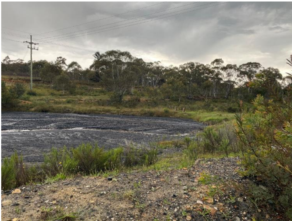
Photo 26: Desilting required in the Stockpile sediment ponds as over 50% of its capacity is covered in fines (refer IMP REC 9).
