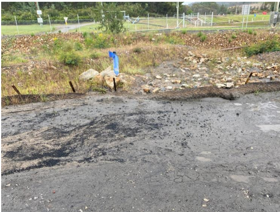
Photo 24: Retention pond requires removal of coal fines blocking filtering through coir logs (refer IMP REC 7).
