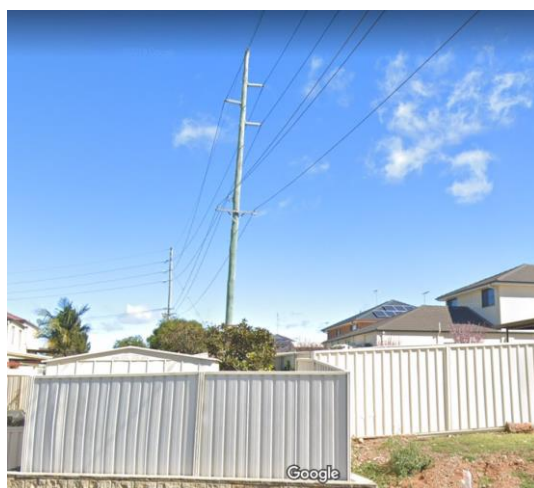
Examples of poor subdivision of easements restricting access and working area around the structures Source: Google Maps Street View.
