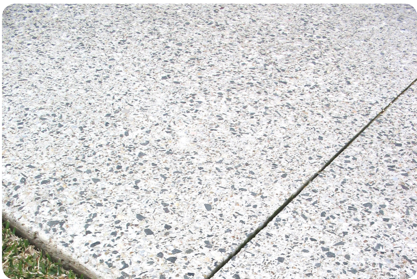
Exposed aggregate insitu concrete
