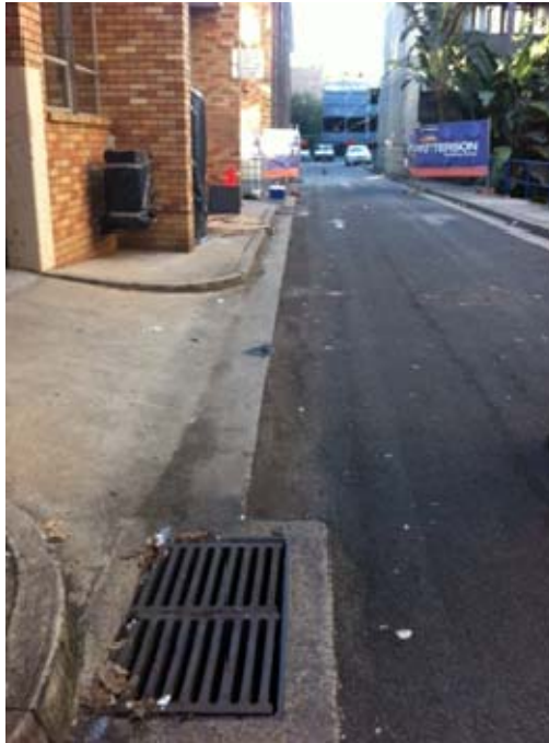
Photo 3: Storm water infrastructure along Willis Lane
