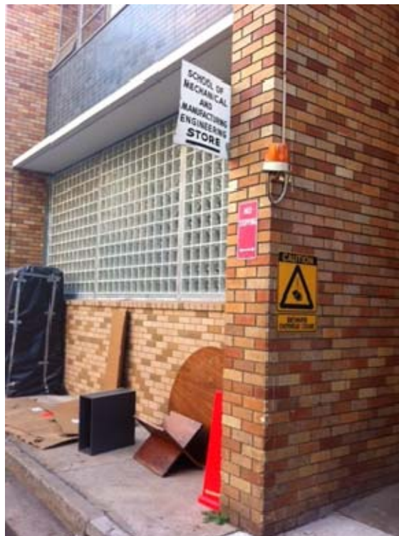
Photo 4: The mechanical and manufacturing engineering store located on the eastern side of Willis Lane.
