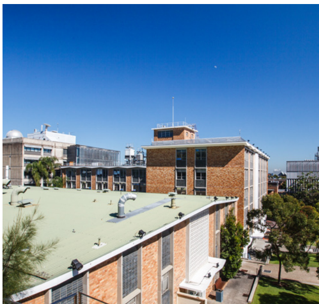
Figure 6 – Mechanical and Manufacturing Precinct looking west (J18 in the foreground, and J17 behind)
