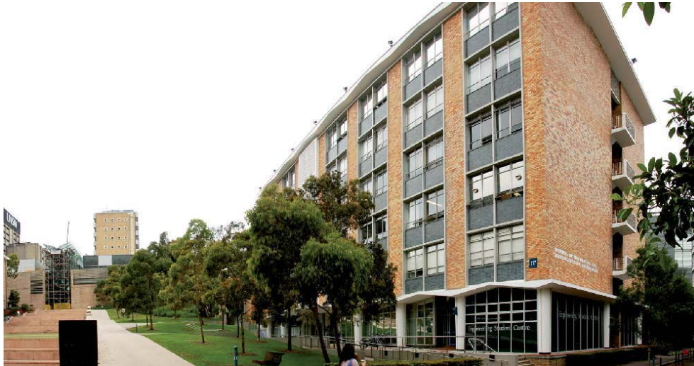
Figure 8 – Building J17 and University mall (looking east).
