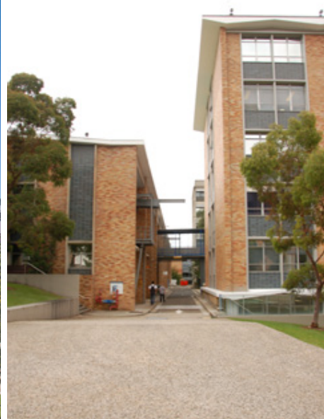
Figure 7 – Willis Lane that runs between buildings J17 and J18 (facing south).
