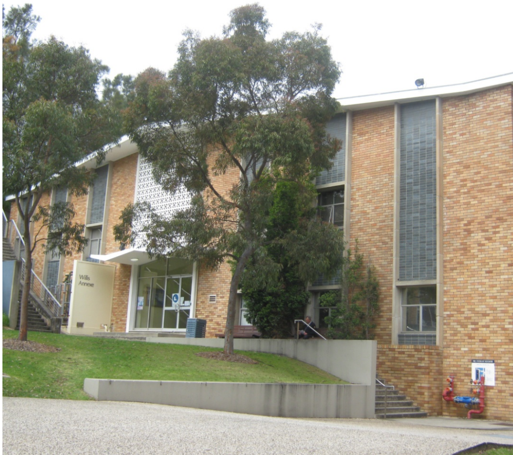
Figure 10 – Northern elevation (frontage) of Building J18.
