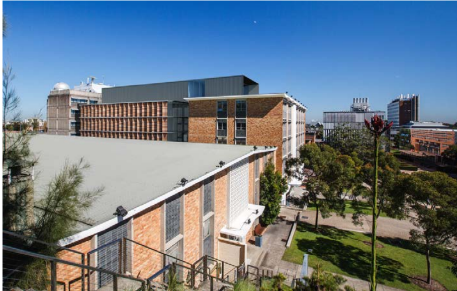
Figure 18 – View of Building J17 and J18 from Willis Street stairs.
