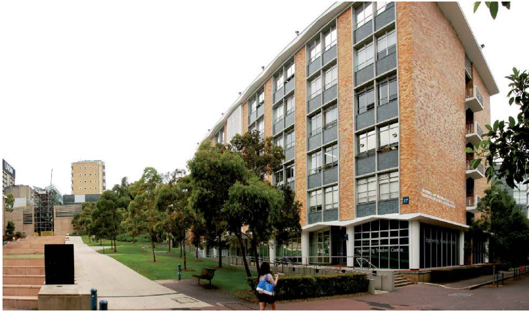
Figure 9 –Building J17 and University Mall
