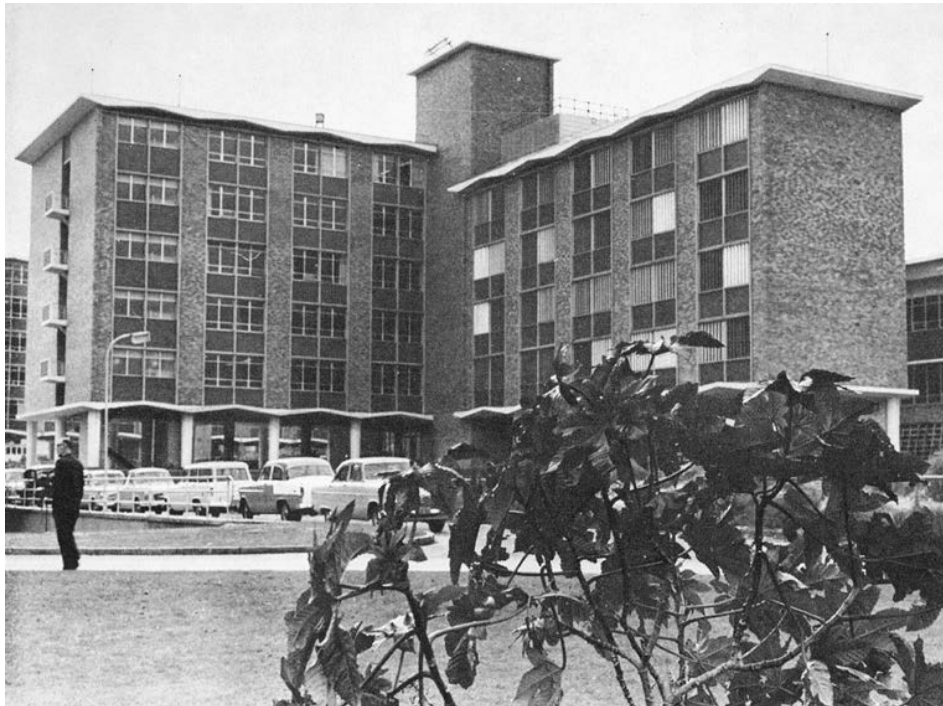
Figure 5 – Building J17 (Mechanical and Manufacturing Engineering Building)
