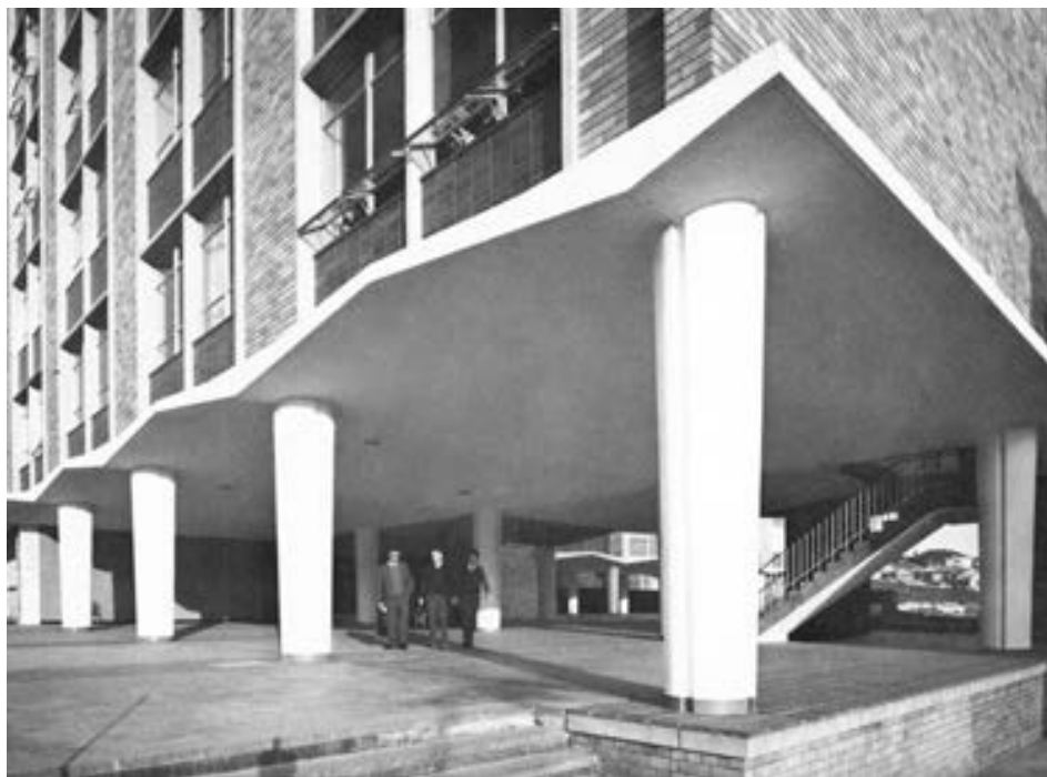
Figure 6 – Historic ground plane of Building J17.
