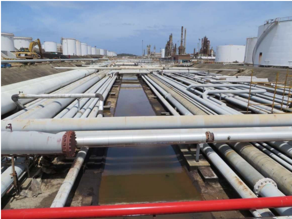
Figure 4-5 Photo of typical pipeway/ open drain section – Main Pipeway (MHL, 2016)
