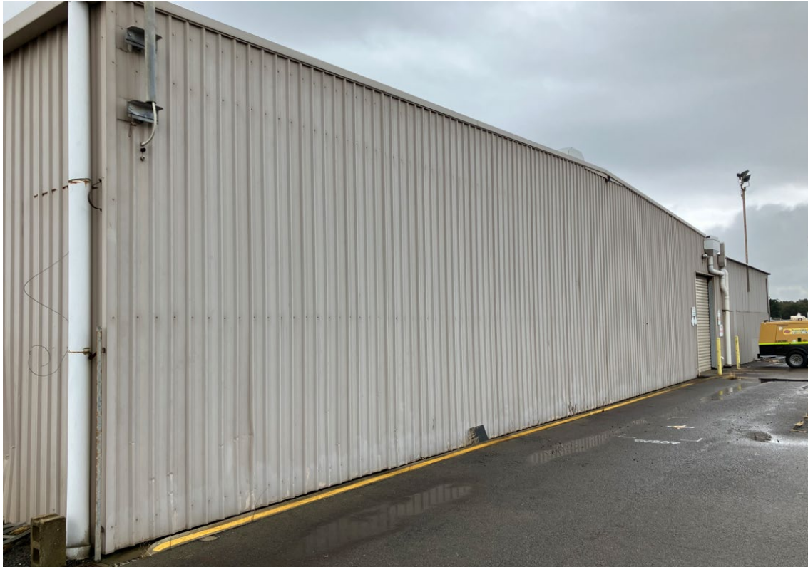
Figure A-3 Storehouse, looking south west (AECOM, 2024)
