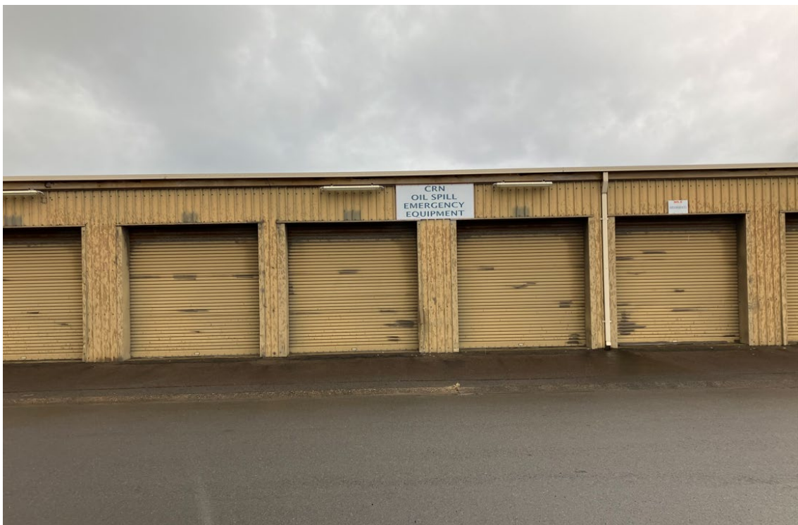
Figure A-2 Oil Spill Room, looking east (AECOM, 2024)
