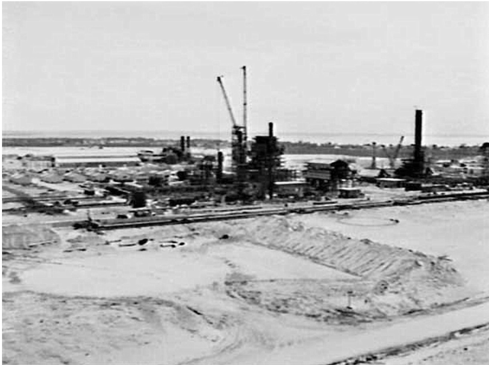
Figure 3-6 Australian Oil Refinery under construction, 1954 (Source: State Library of NSW, Call Number: Australian Photographic Agency – 42956)
