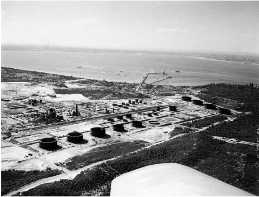
Figure 3-8 Aerial view of construction of the Australian Oil Refinery, 1955, with wharf in background (Source: State Library of NSW, Call number: Australian Photographic Agency – 00036)
