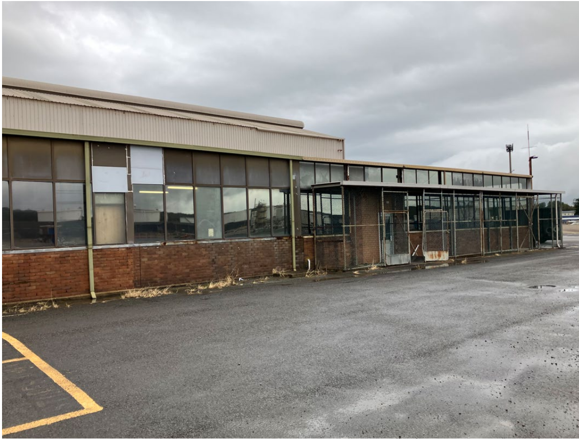
Figure A-7 Warehouse, looking northwest (AECOM, 2024)
