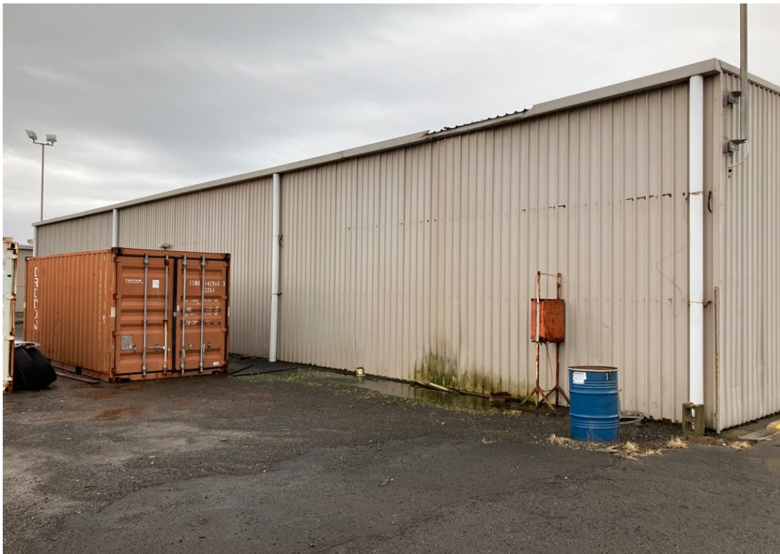
Figure A-4 Storehouse, looking southwest (AECOM, 2024)
