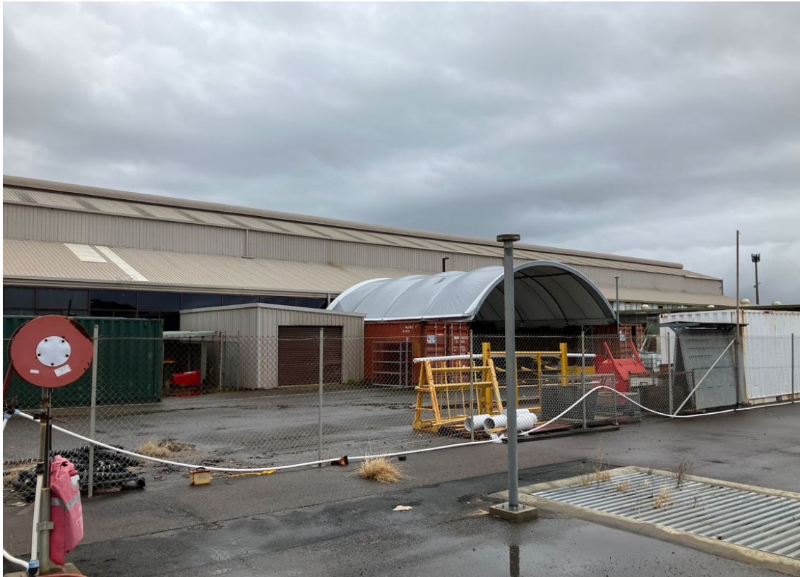
Figure A-5 Warehouse, looking southeast (AECOM, 2024)
