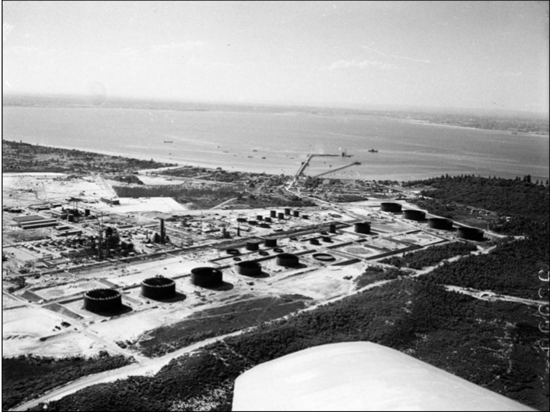
Plate 5-7 Aerial view of construction of the Australian Oil Refinery, 1955, with wharf in the background (Source: State Library of NSW, Australian Photographic Agency – 00036)
