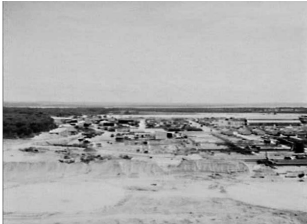
Plate 5-2 Photo of the refinery under construction on 25 September 1954 view west (source: Jack Hickson, State Library of NSW)
