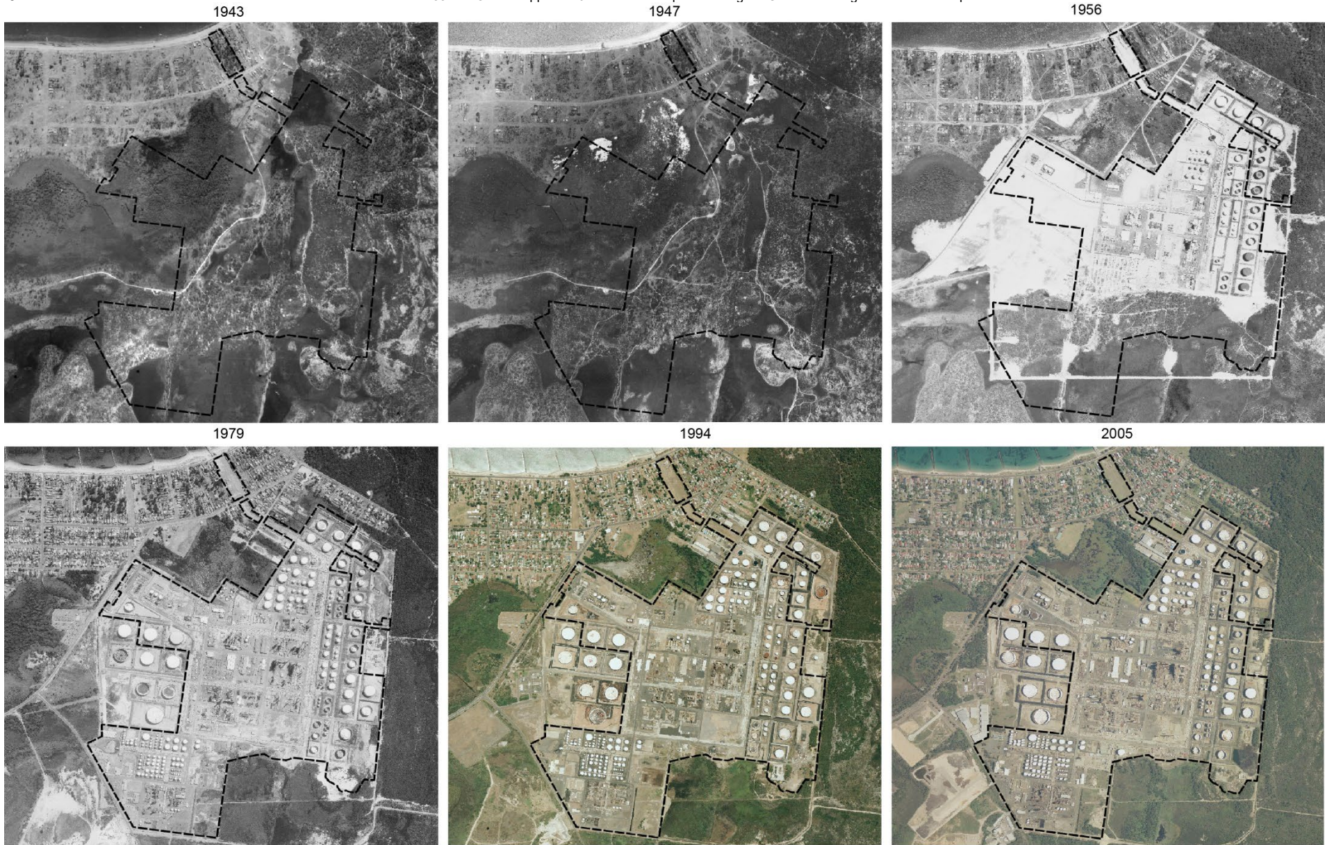
Figure 5-13 Aerial photographs of the Project Area (Source: Land and Property Information NSW)
