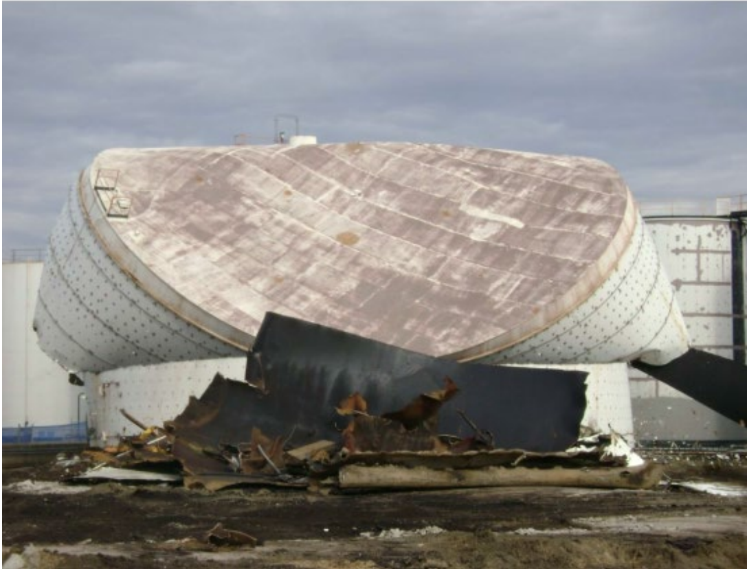
Figure C-6 Excavator/ shear part 3
