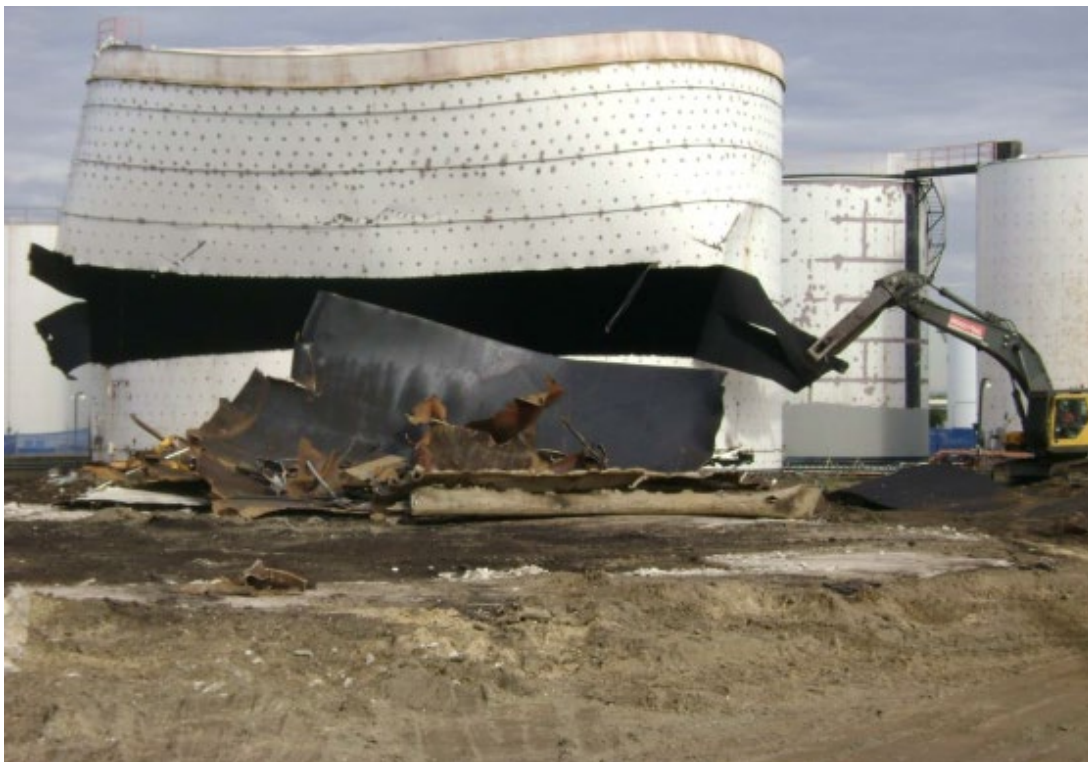
Figure C-5 Excavator/ shear part 2
