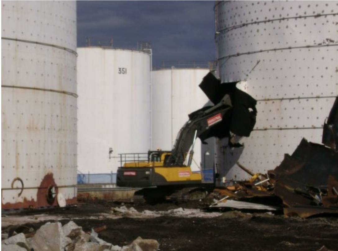
Figure C-4 Excavator/ shear Part 1
