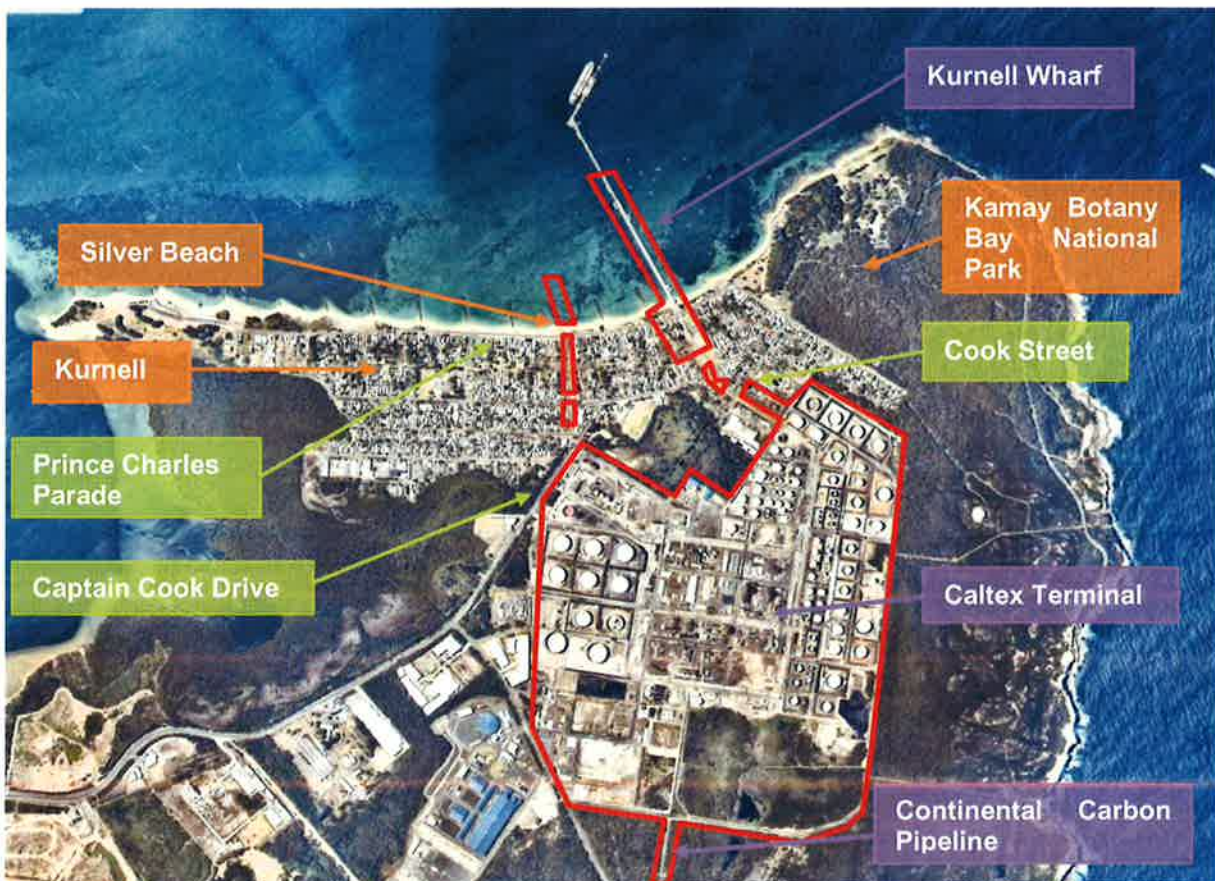
Figure 1: Site Context and Surrounding Uses
