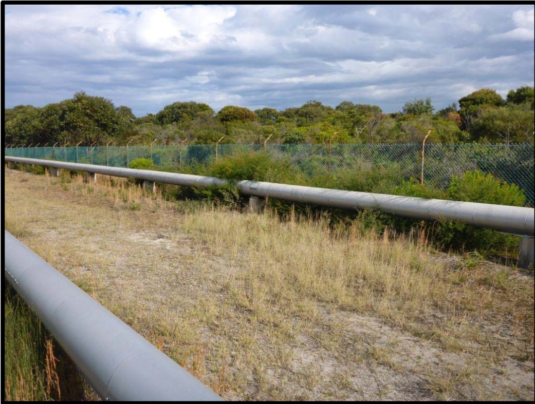
Plate 3: Continental Pipeline - southern section showing modified vegetation within pipeline easement
