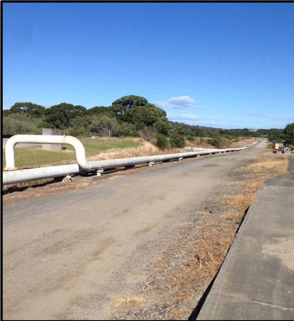
Plate 2: Continental Pipeline – northern section looking south from Kurnell Terminal
