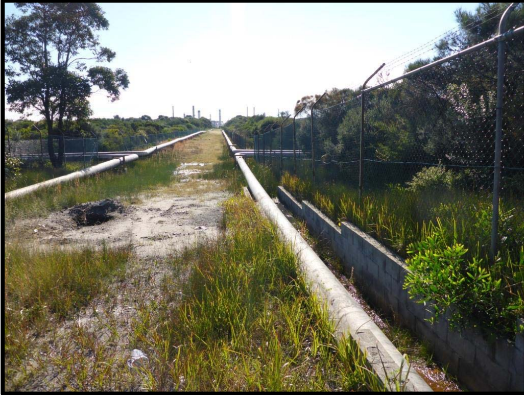
Plate 1: Continental Pipeline – central section looking north towards Kurnell Terminal
