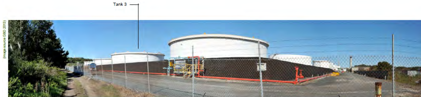
Photo Location K8 - Existing view toward Tank 3 from access track south west and parallel to Reserve Road
