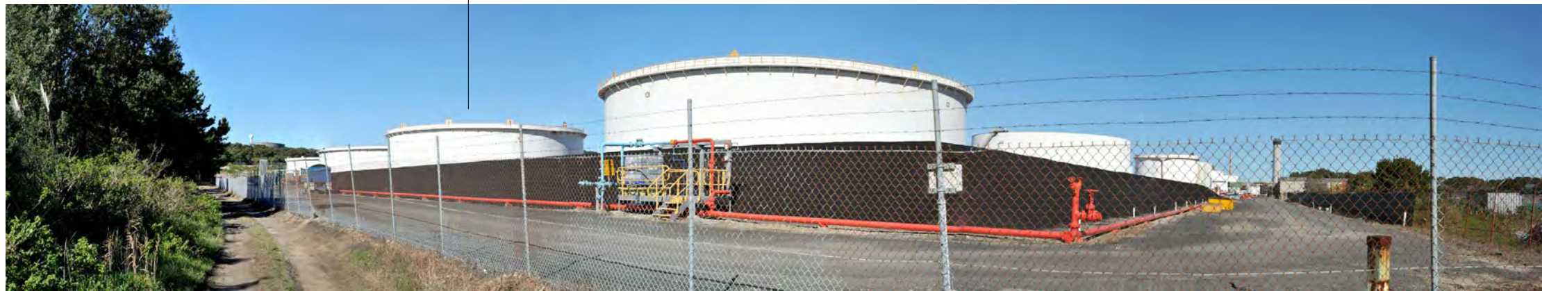
Photo Location K8 - Access track south west and parallel to Reserve Road
